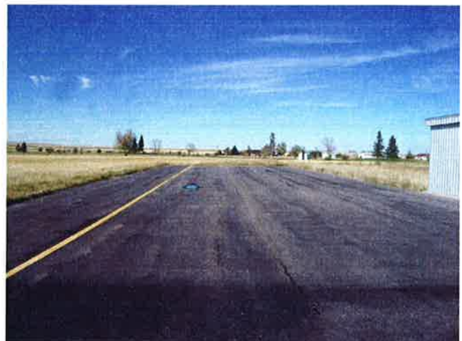
T-4 , Hangar area overview
