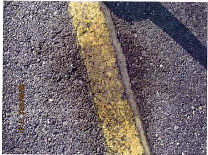
T-2, Surface detail with oil spillage
