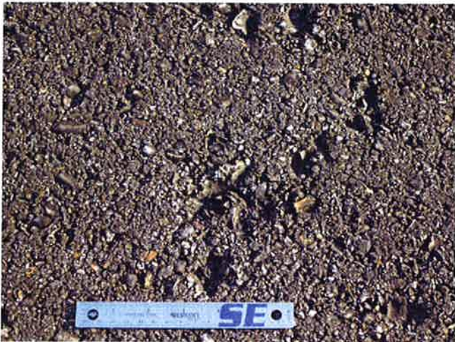
R-1 , Surface detail with raveling
