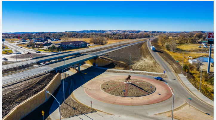
Completed Broadus Interchange roundabout in Miles City, Mont.
