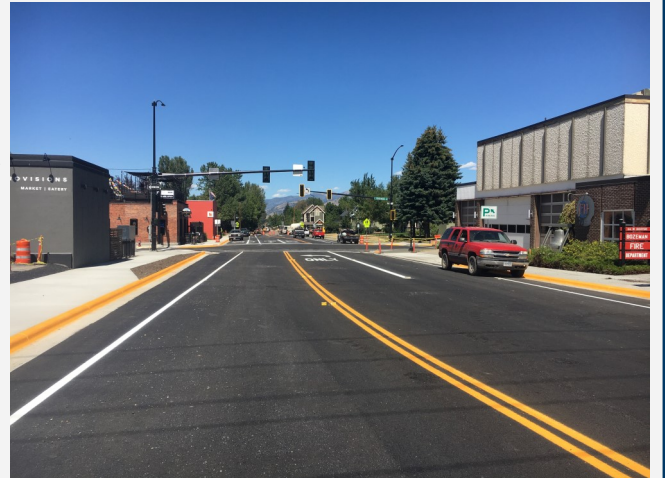
Construction in 2020 on Rouse Avenue in Bozeman, Mont.
