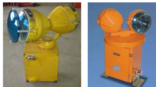
The Browning airport had their rotating beacon (left) replaced with a newer rotating beacon (right).
