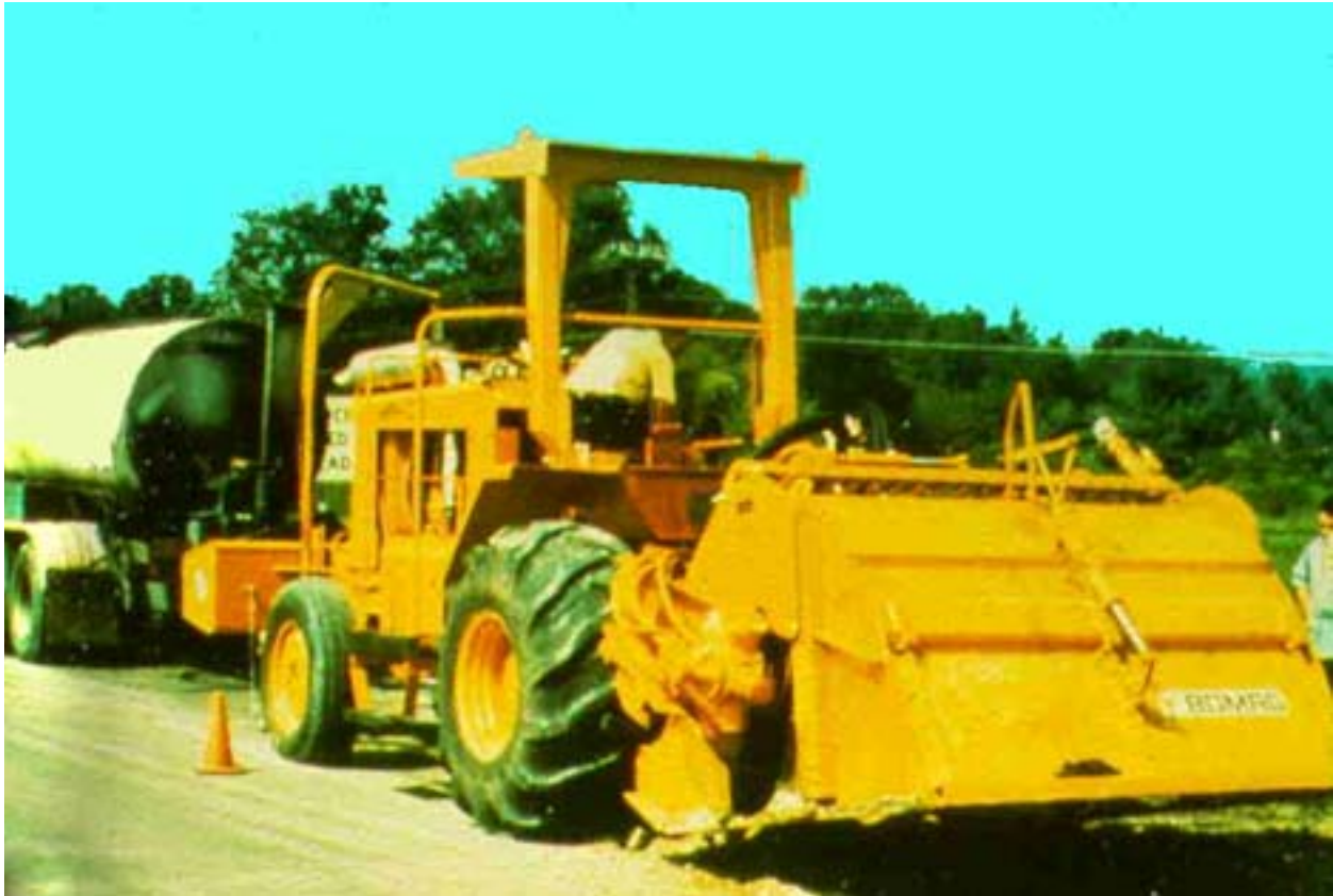
Figure 9-6 Asphalt Pavement Reclaiming Machine Adding Asphalt Emulsion
