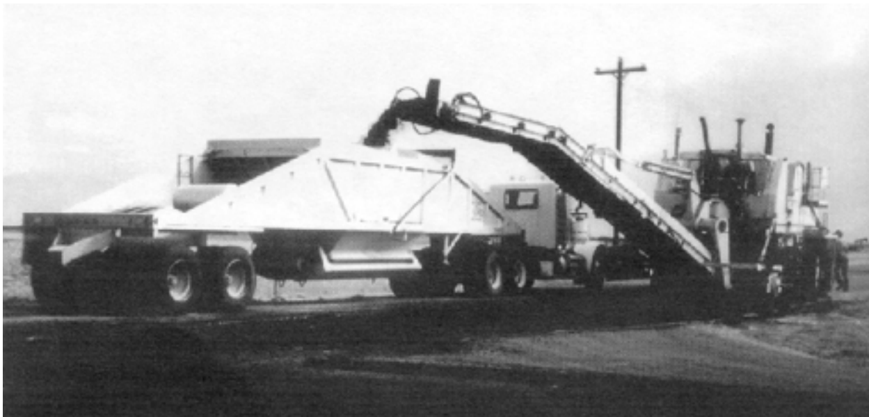
Figure 9-3 Cold Planing/Milling Machine Removing Asphalt Pavement
