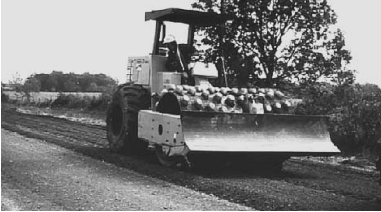
Figure 12-6: Compaction of FDR mix
