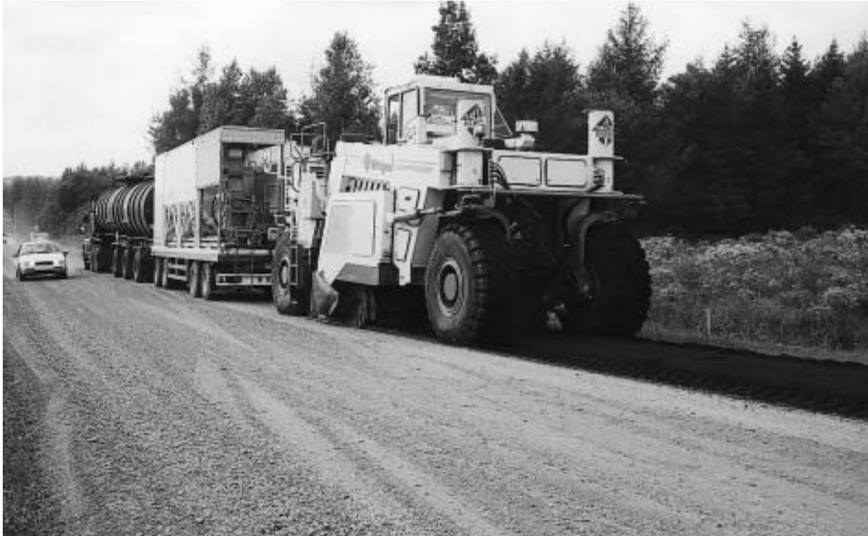
Figure 11-6: Bituminous stabilization operation with cement slurry (combination stabilization)
