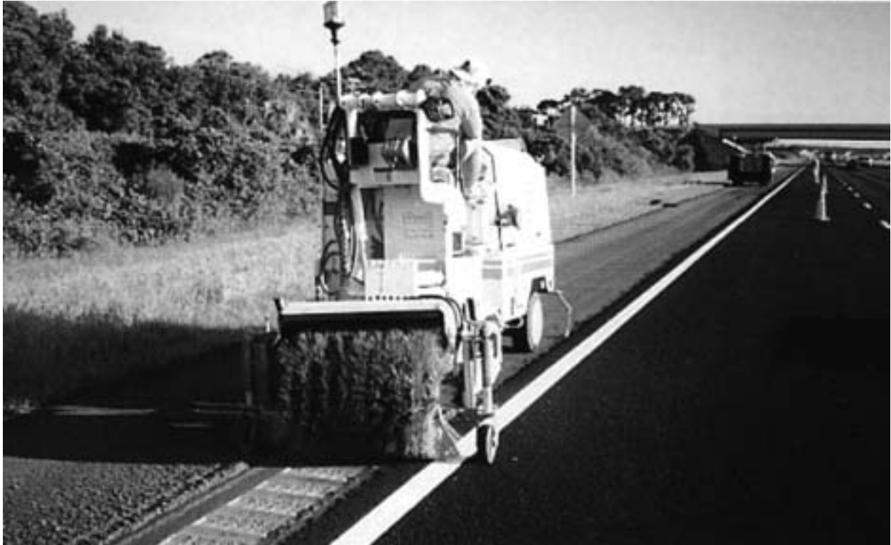
Figure 8-12: Installation of longitudinal rumble strips
