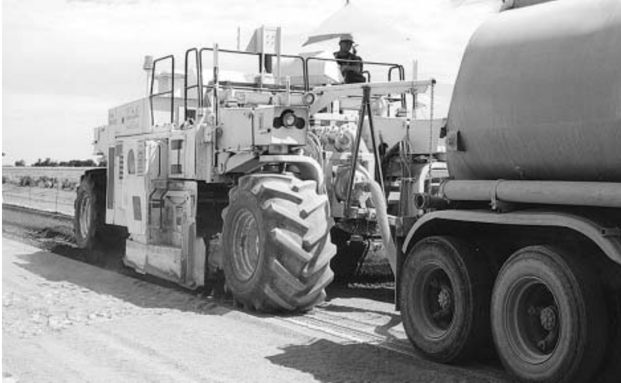
Figure 11-2: Chemical stabilization on rural roadway
