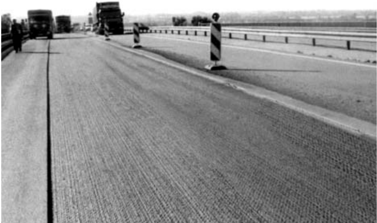
Figure 8-11: CP surface texture produced with a micro milling drum
