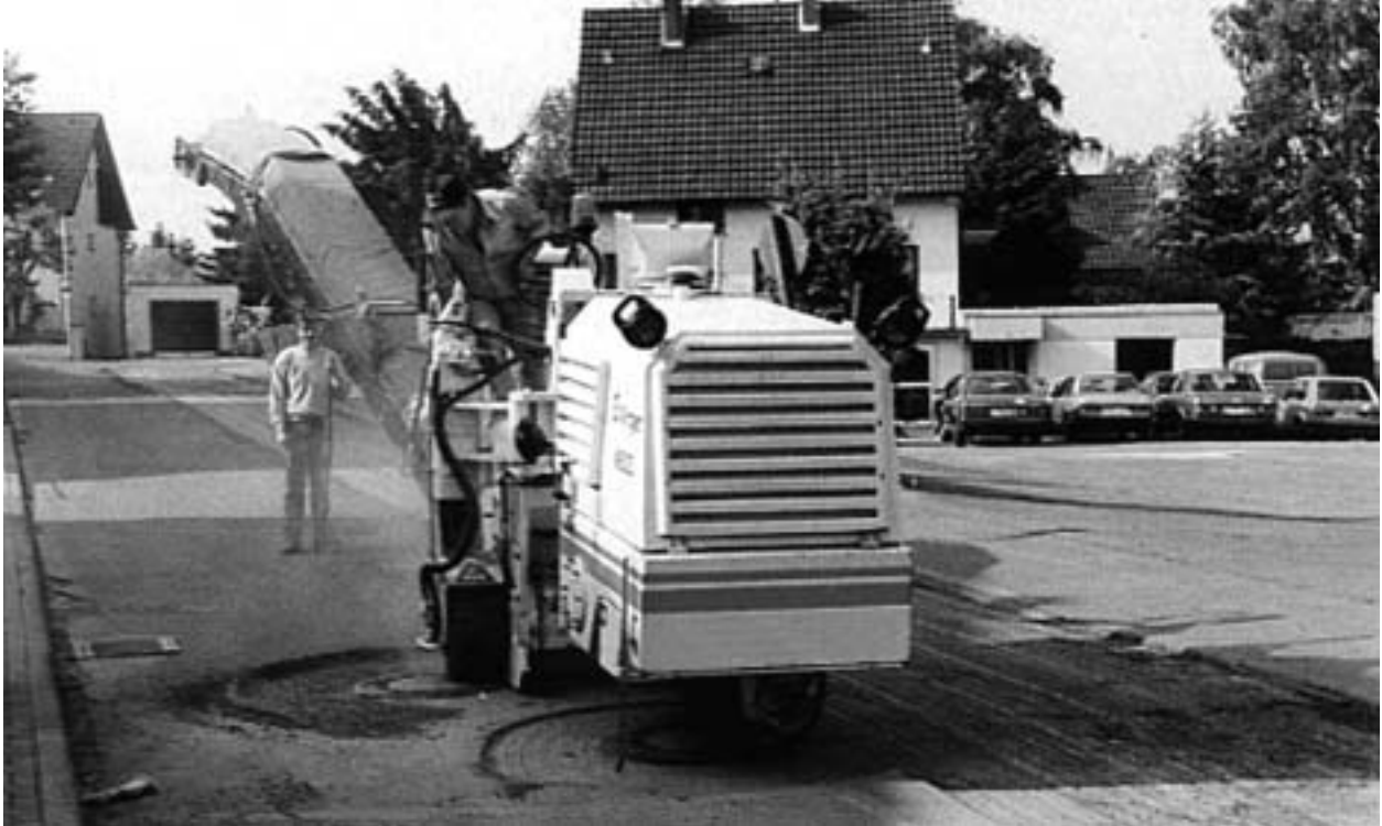
Figure 8-1: Mini cold planer working around a manhole
