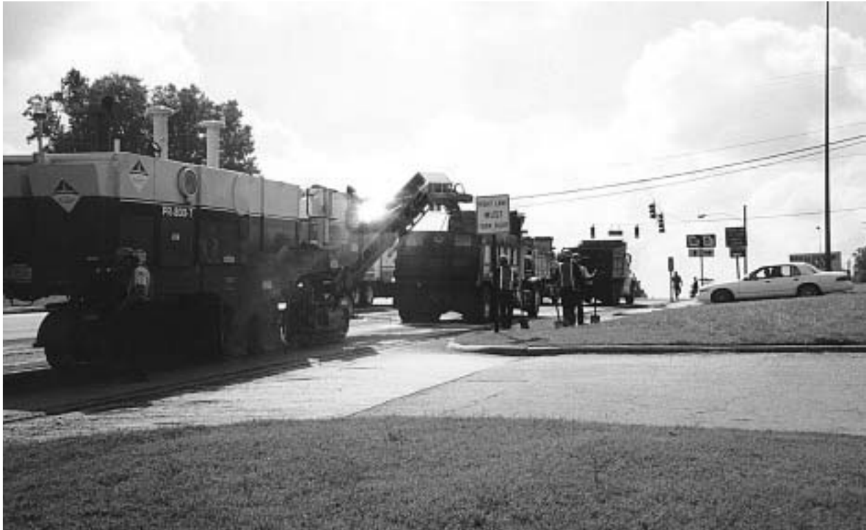
Figure 8-4: Cold planer milling urban intersection
