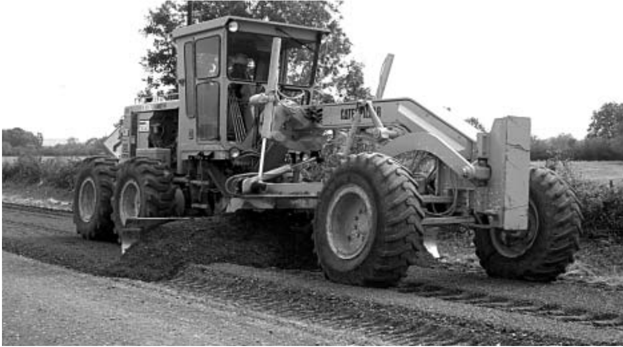
Figure 12-5: Motor grader blading FDR mix
