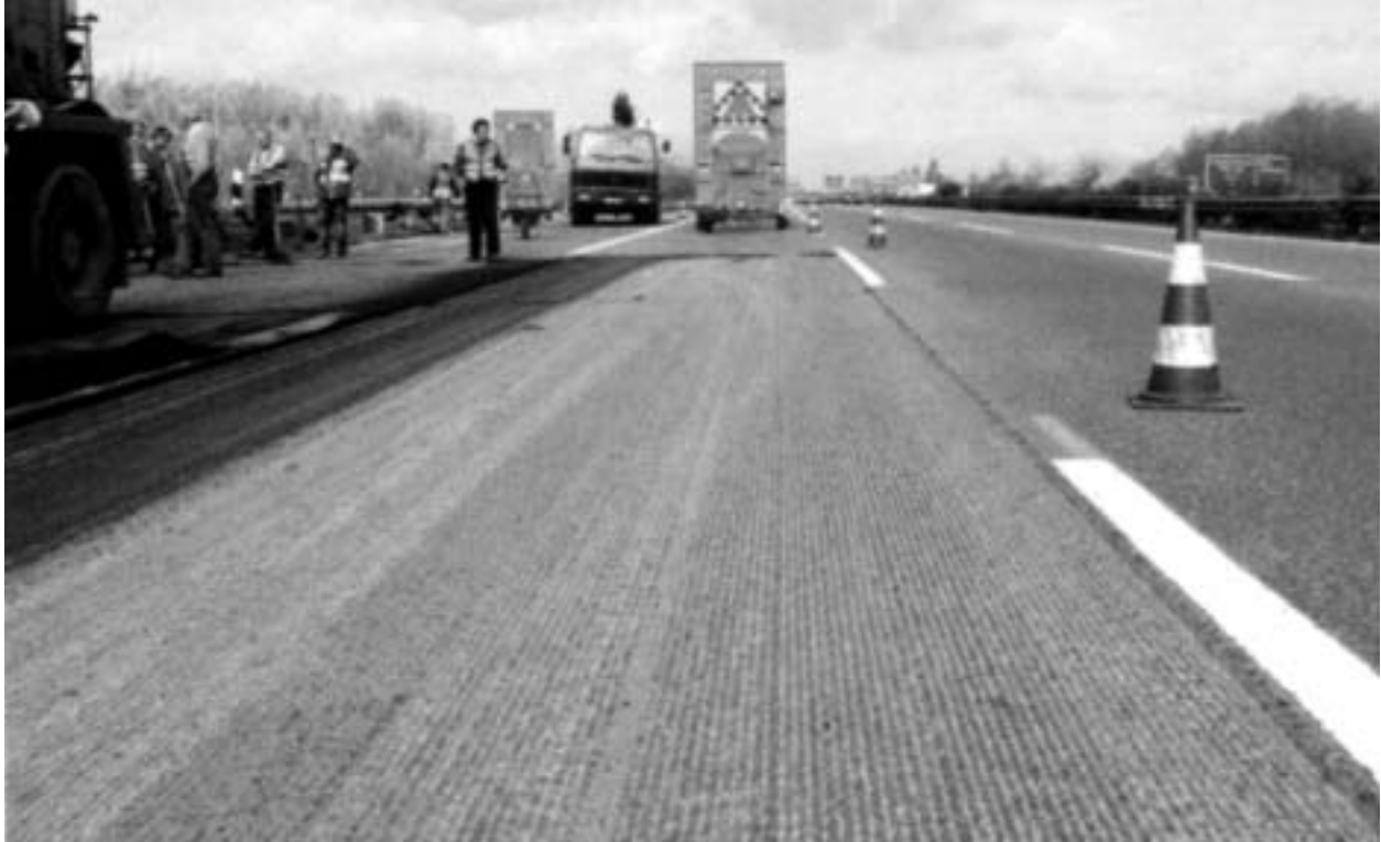
Figure 8-10: CP surface texture produced with a conventional milling drum
