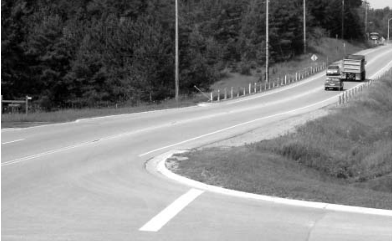
Figure 14-2: Completed CIR Project with a Hot Mix Overlay
