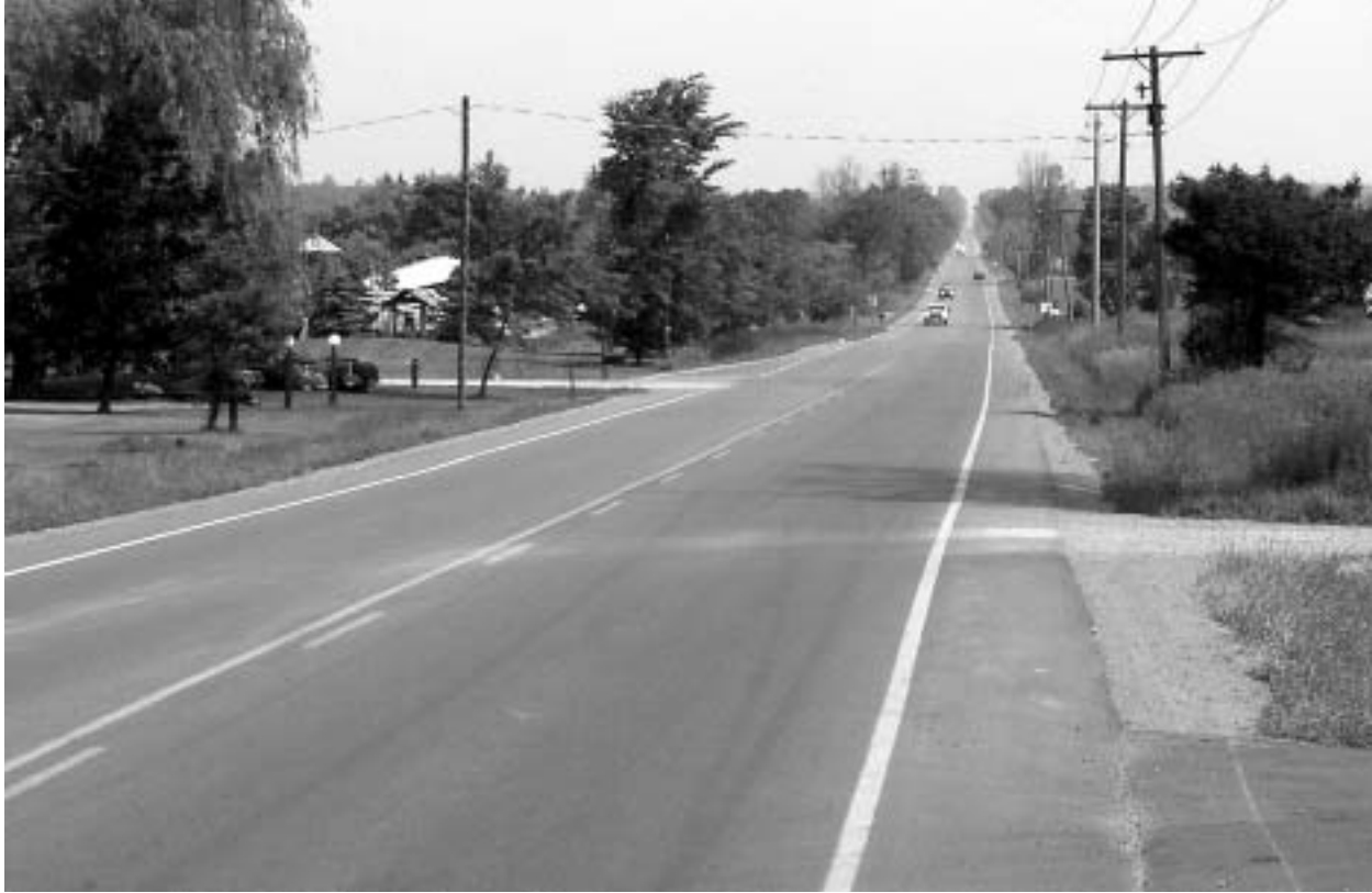
Figure 13-1: Completed FDR with Hot Mix Overlay
