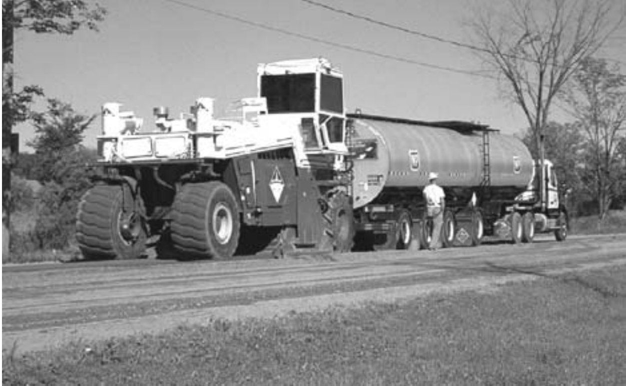
Figure 11-4: Foamed asphalt operation
