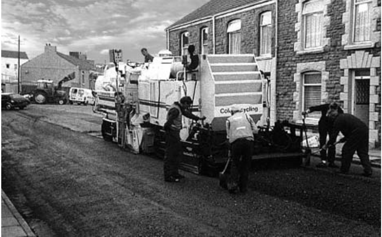
Figure 1-18: Single unit CIR train
