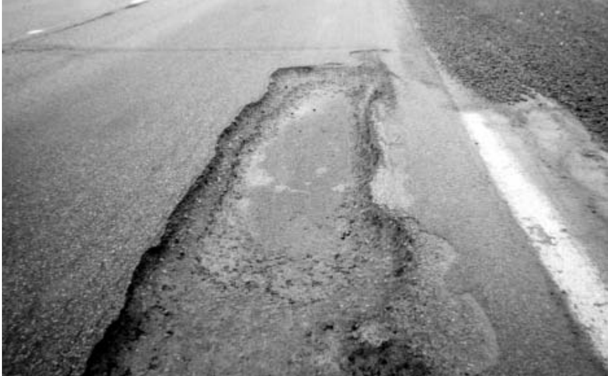
Figure 3-1: Pothole Pavement
