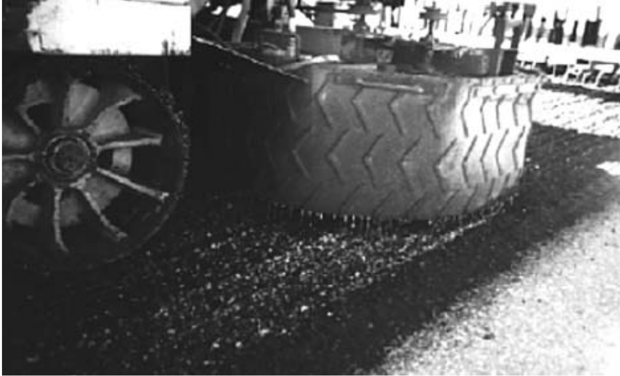
Figure 6-4: Recycling agent addition
