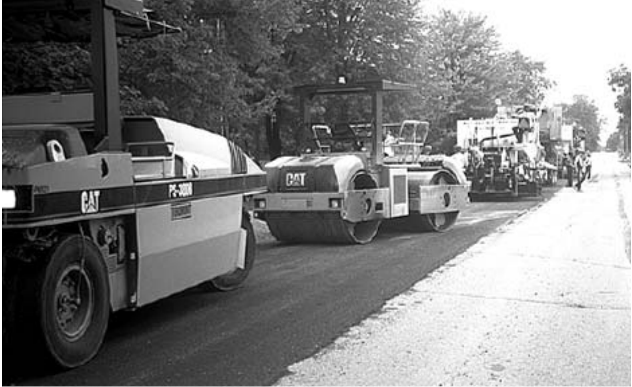
Figure 1-21: CIR compaction
