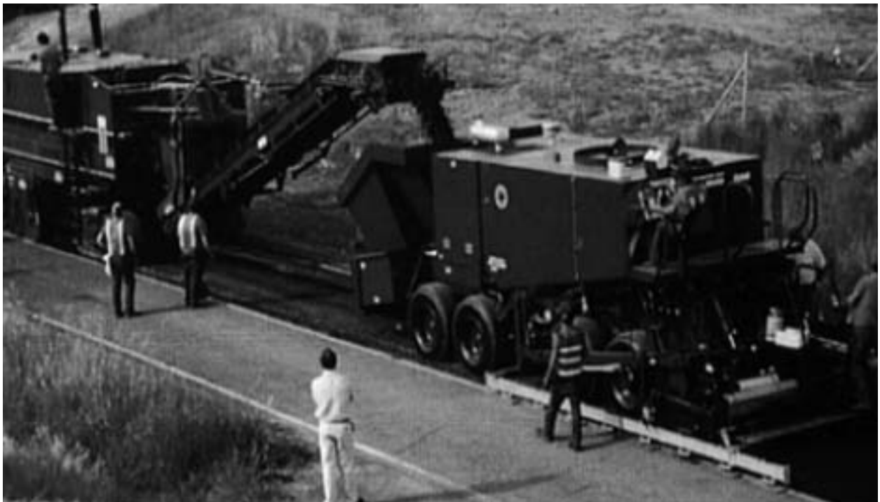
Figure 1-19: Two-unit CIR train
