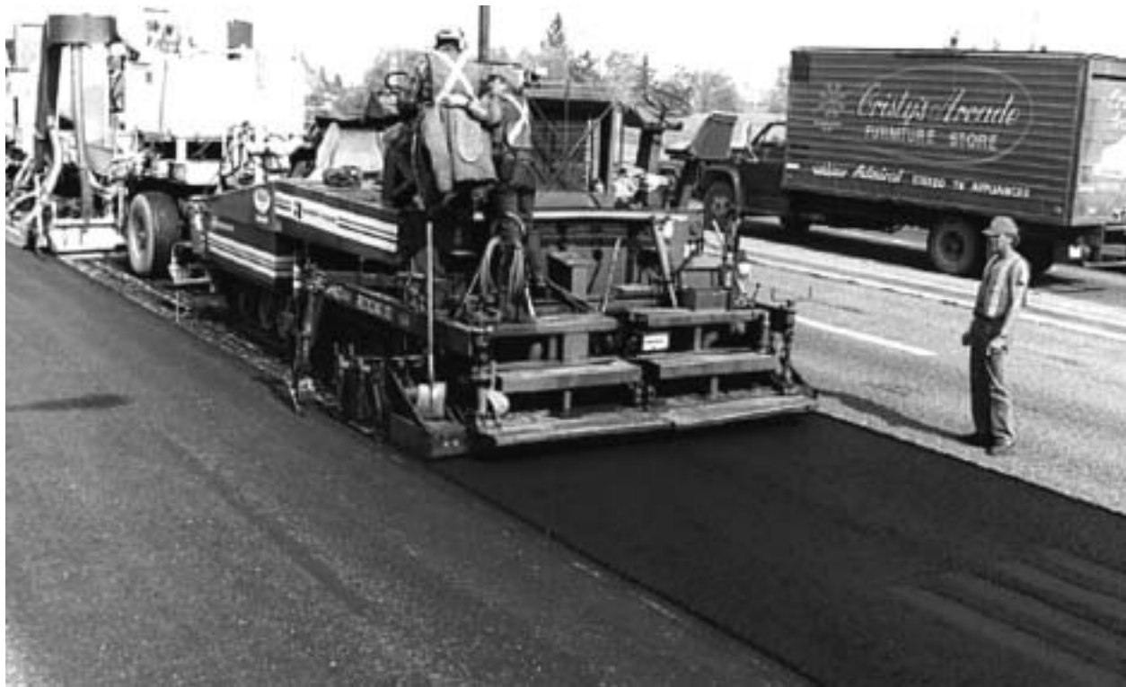
Figure 6-17: Conventional HMA paver placing recycled mix
