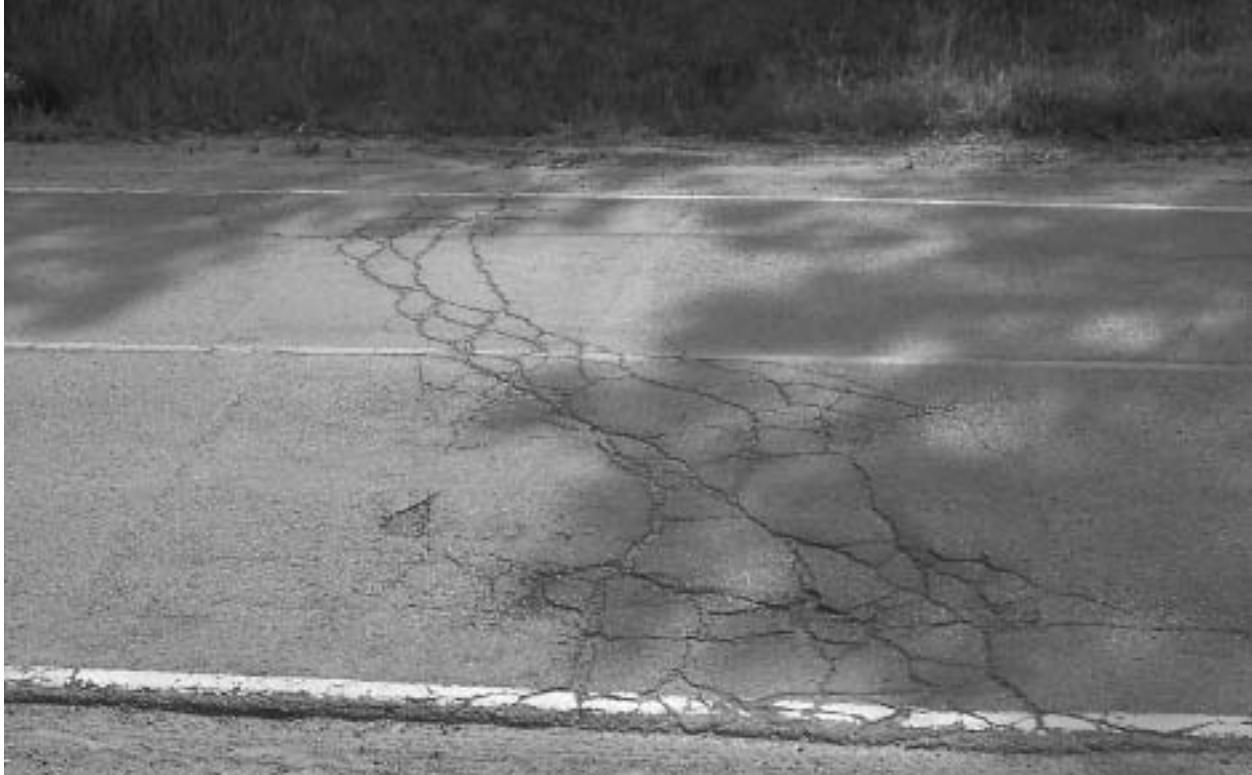
Figure 3-2: Cracking Distress
