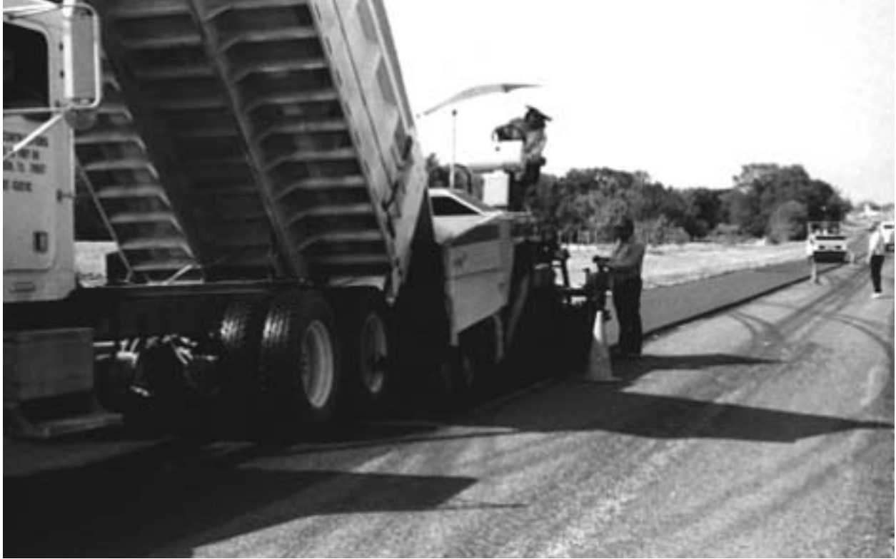
Figure 1-24: CCPR mix placement
