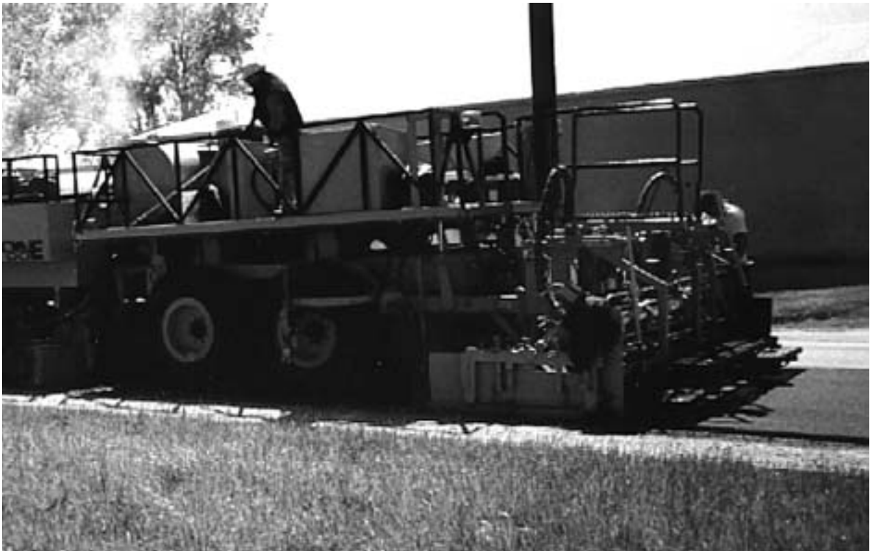
Figure 6-16: Remixing unit and integrated screed
