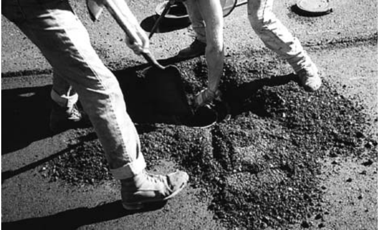
Figure 6-18: Raising water valve after remixing
