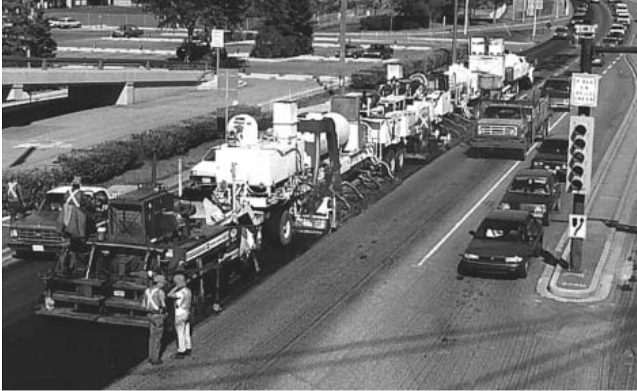
Figure 1-10: HIR Remixing train
