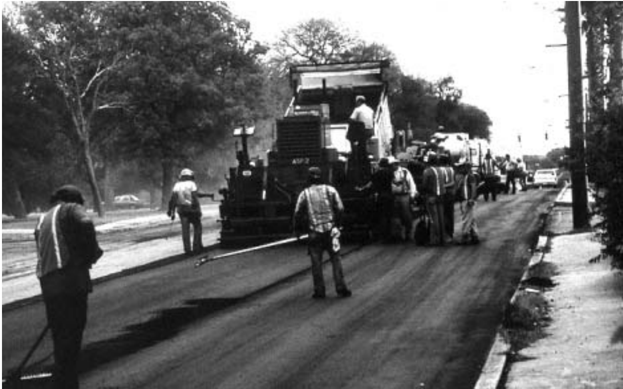
Figure 1-13: Multiple pass repaving
