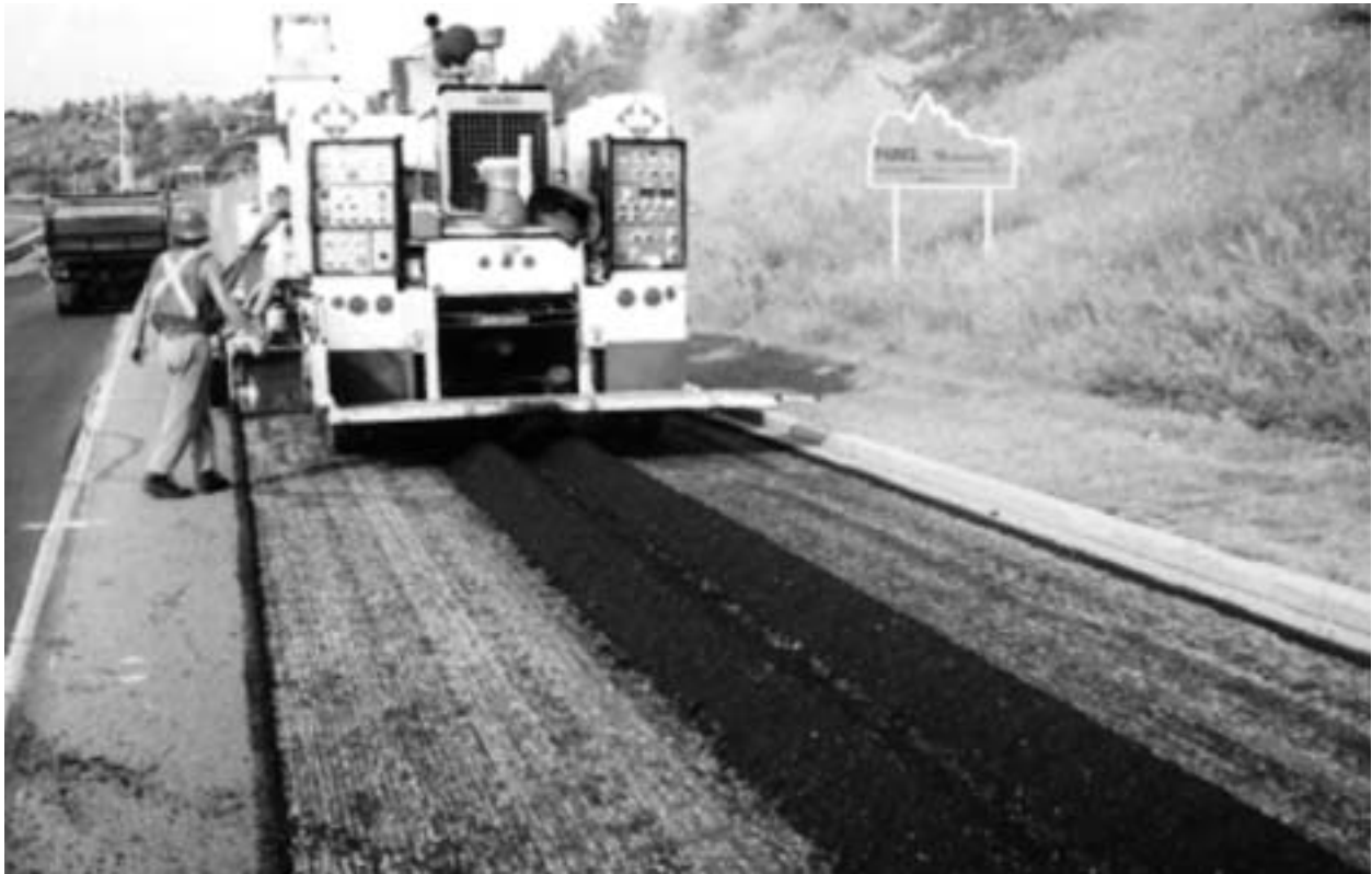
Figure 1-12: Multiple stage Remixing with windrow of scarified material
