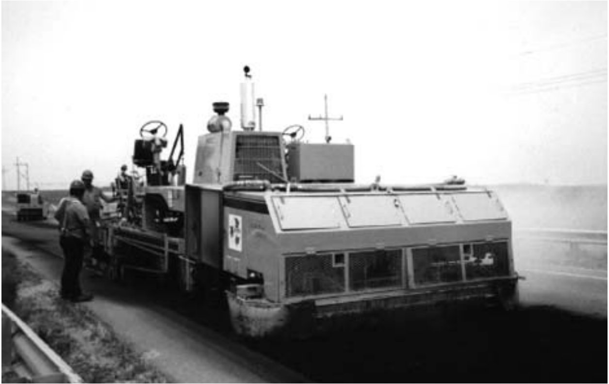
Figure 6-5: Recycling agent addition, mixing, and paving unit
