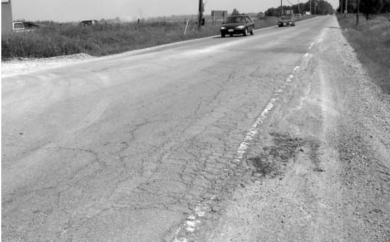
Figure 2-4: Candidate Road for Rehabilitation Treatment
