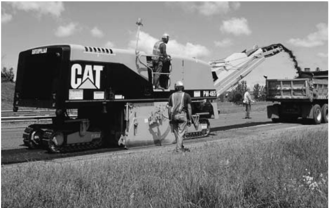
Figure 1-4: Half-lane cold planing machine
