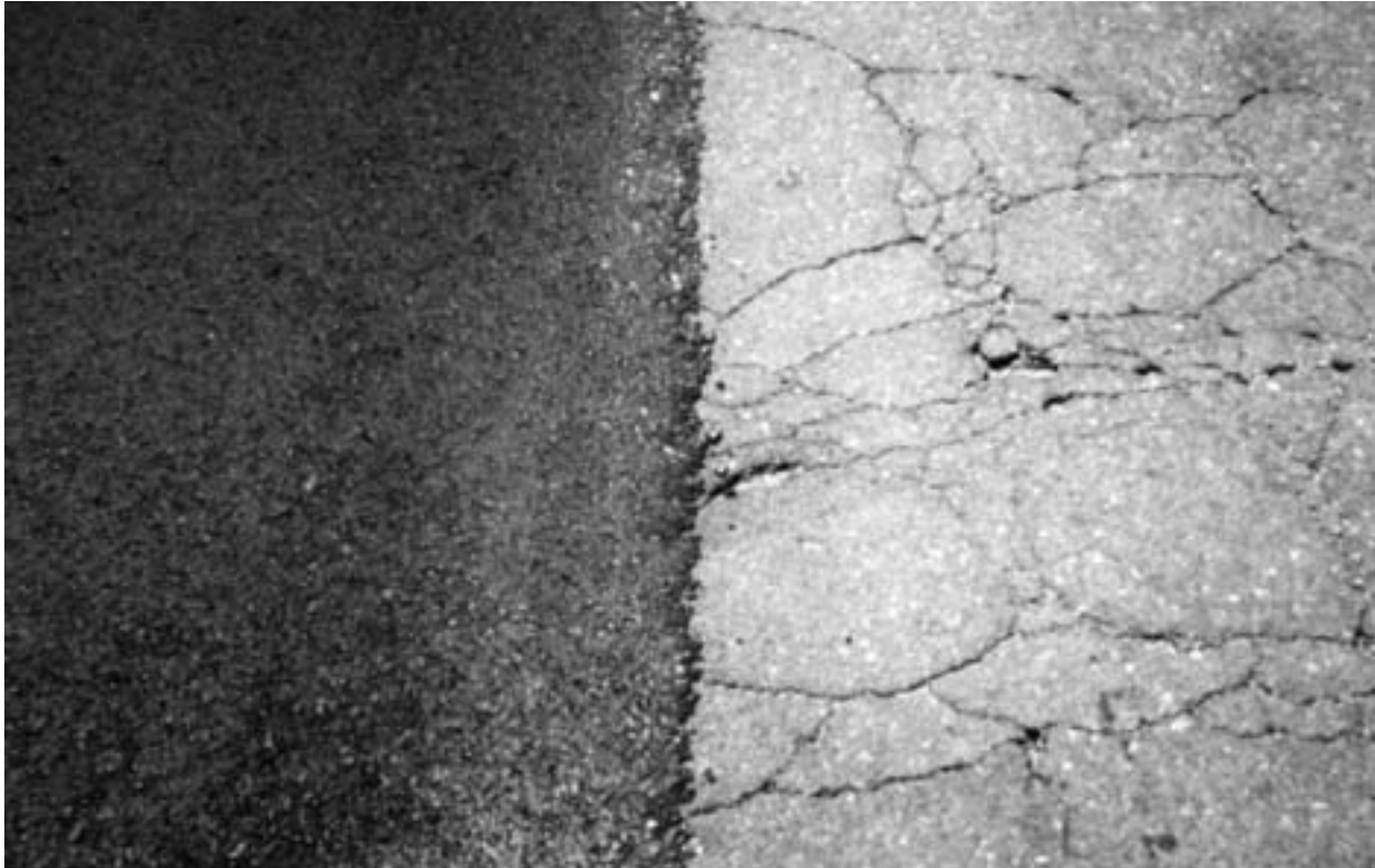
Figure 6-10: Surface Recycling before and after
