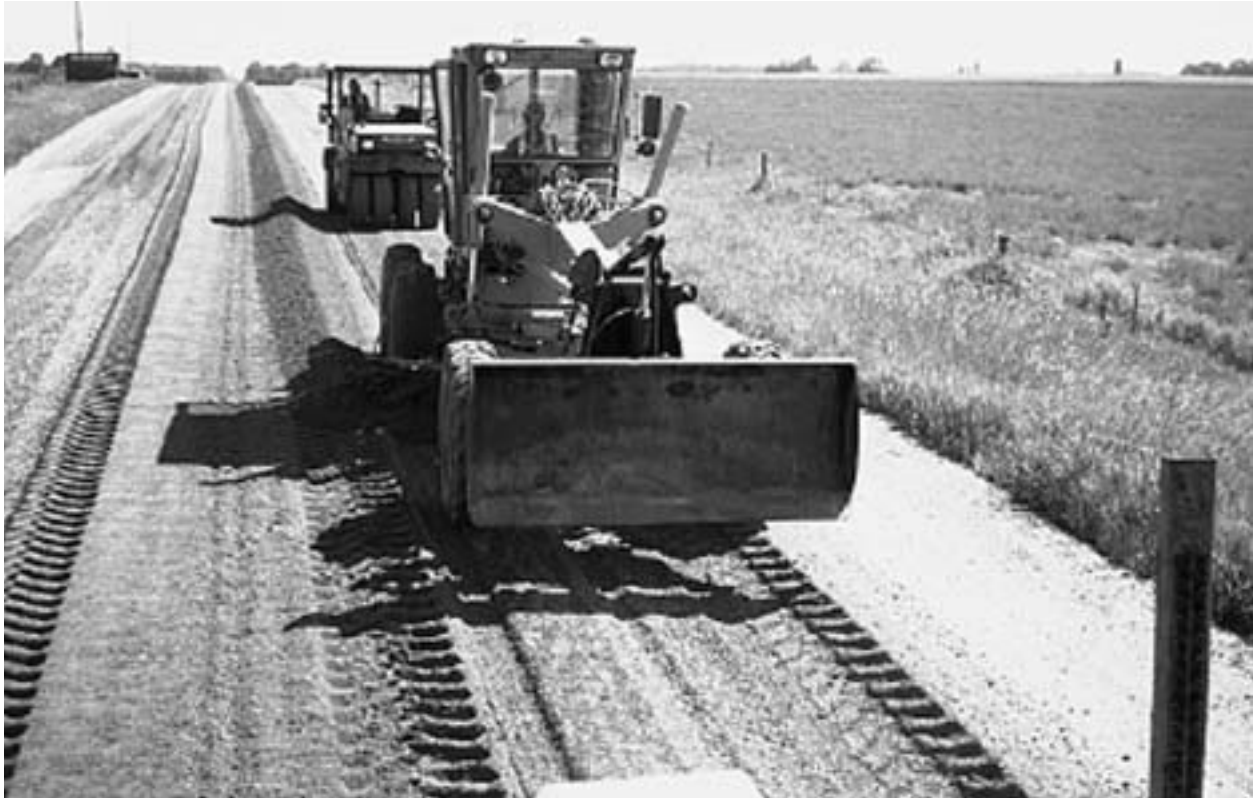
Figure 1-17: Initial shaping with motor grader and compaction
