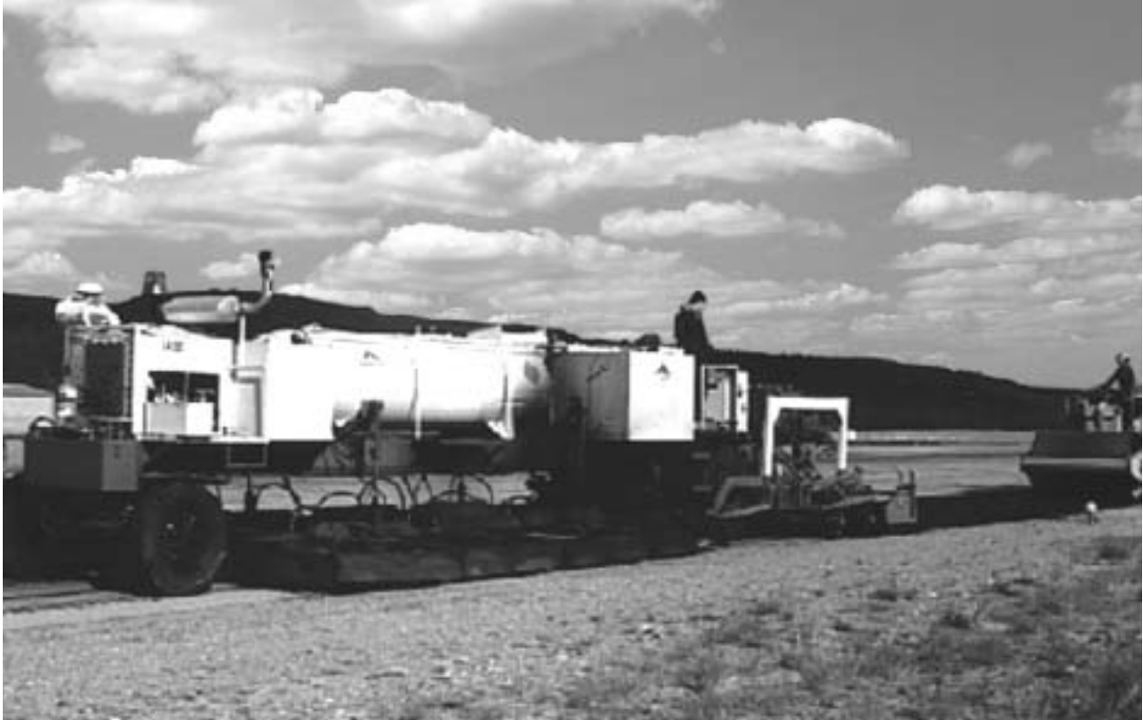
Figure 6-7: Free floating screed on scarification unit
