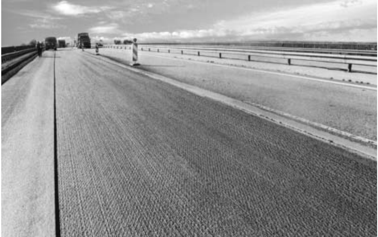
Figure 1-3: Milled pavement surface texture improve friction numbers
