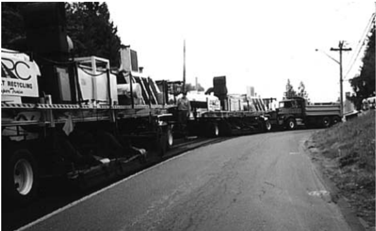
Figure 6-12: Multiple stage Remixing train
