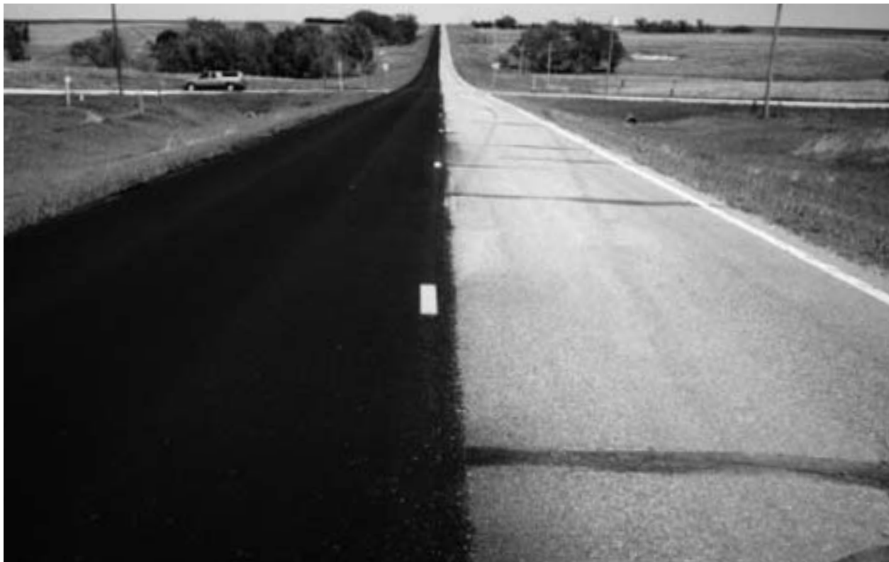
Figure 6-9: Surface Recycling before and after
