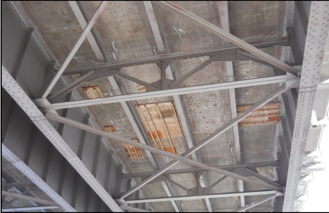
Photo 24. Cracking concrete with efflorescence and concrete deck patching with formwork left in place on the Madison Street Bridge.
