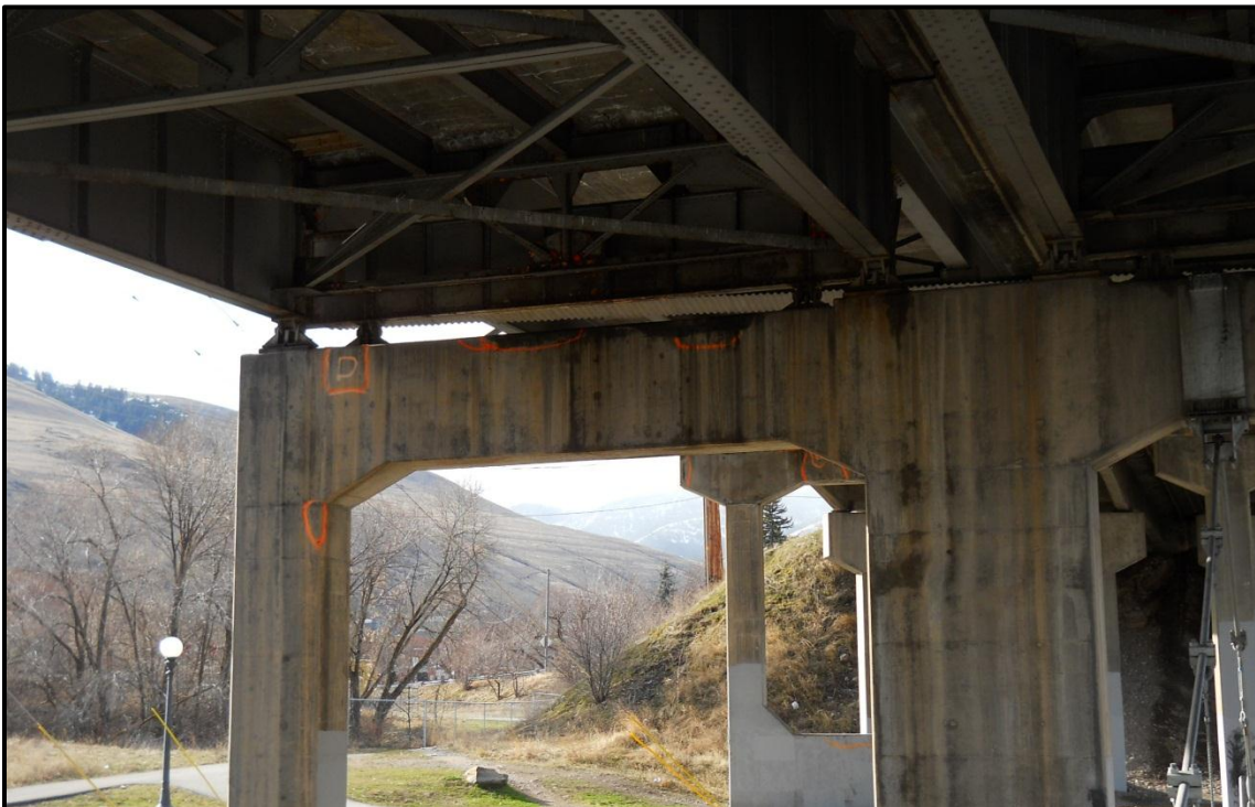
Photo 21. Corroded steel and concrete delamination on a Madison Street Bridge bent.
