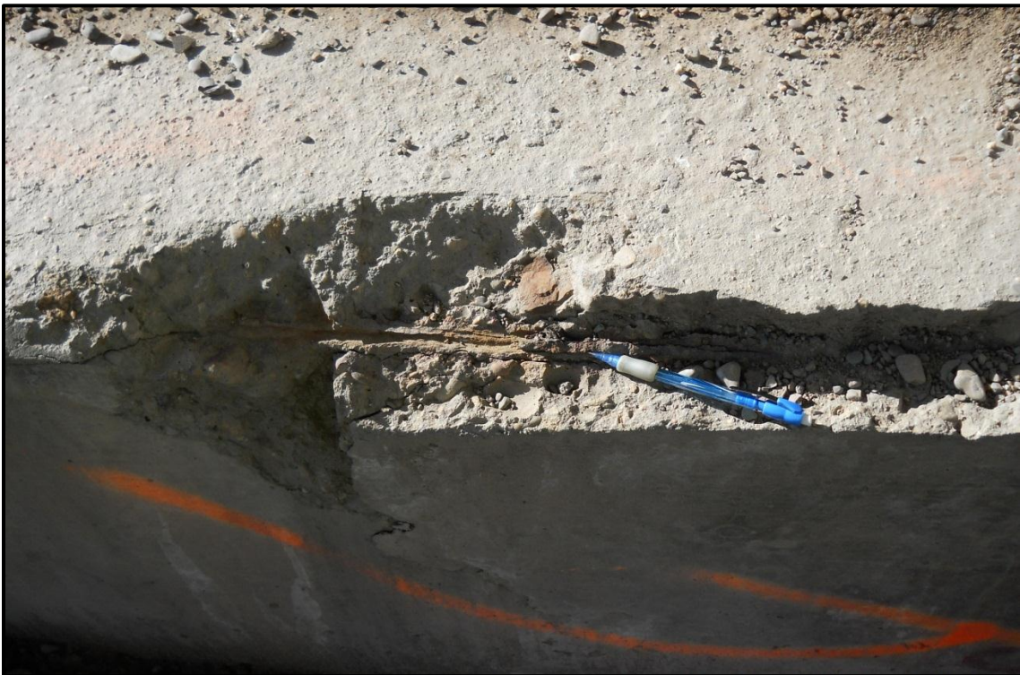
Photo 25. Delaminated/spalled concrete and corroded rebar on the Madison Street Bridge.
