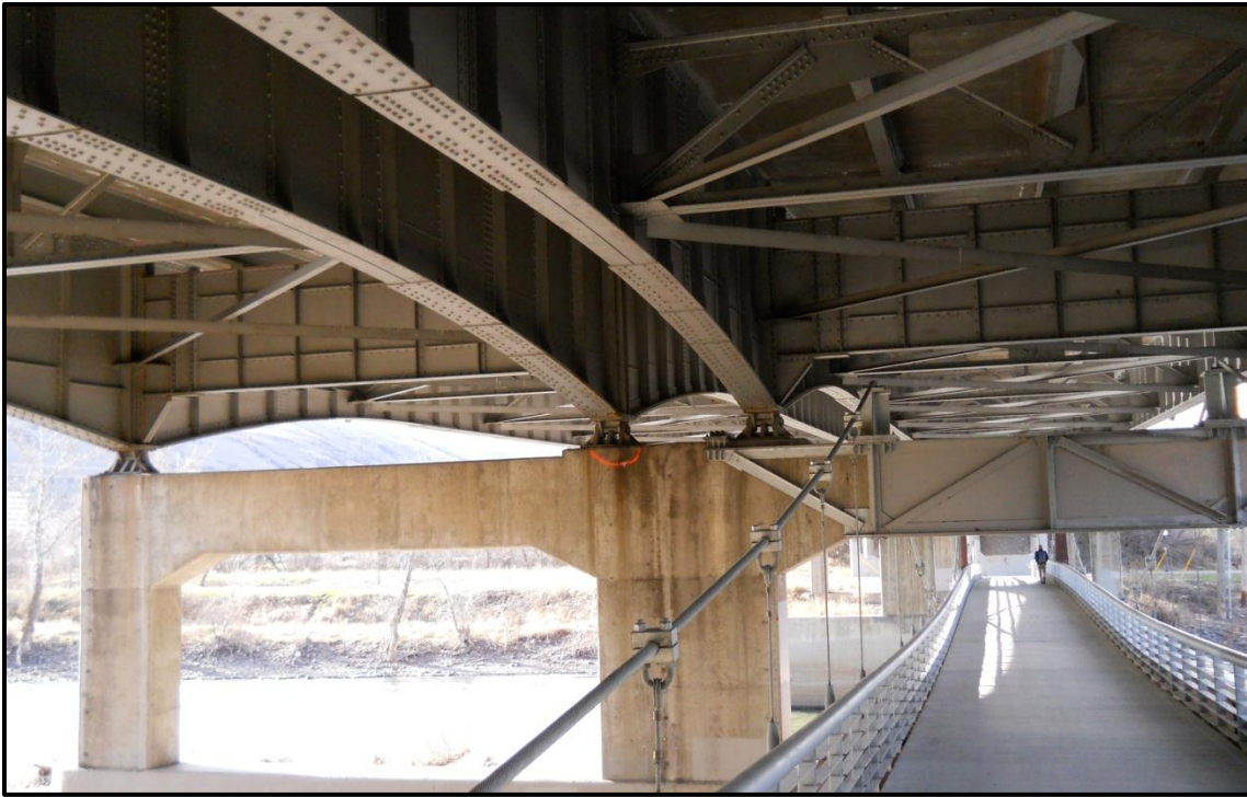
Photo 18. Orange paint delineating steel corrosion and concrete delamination on the Madison Street Bridge.
