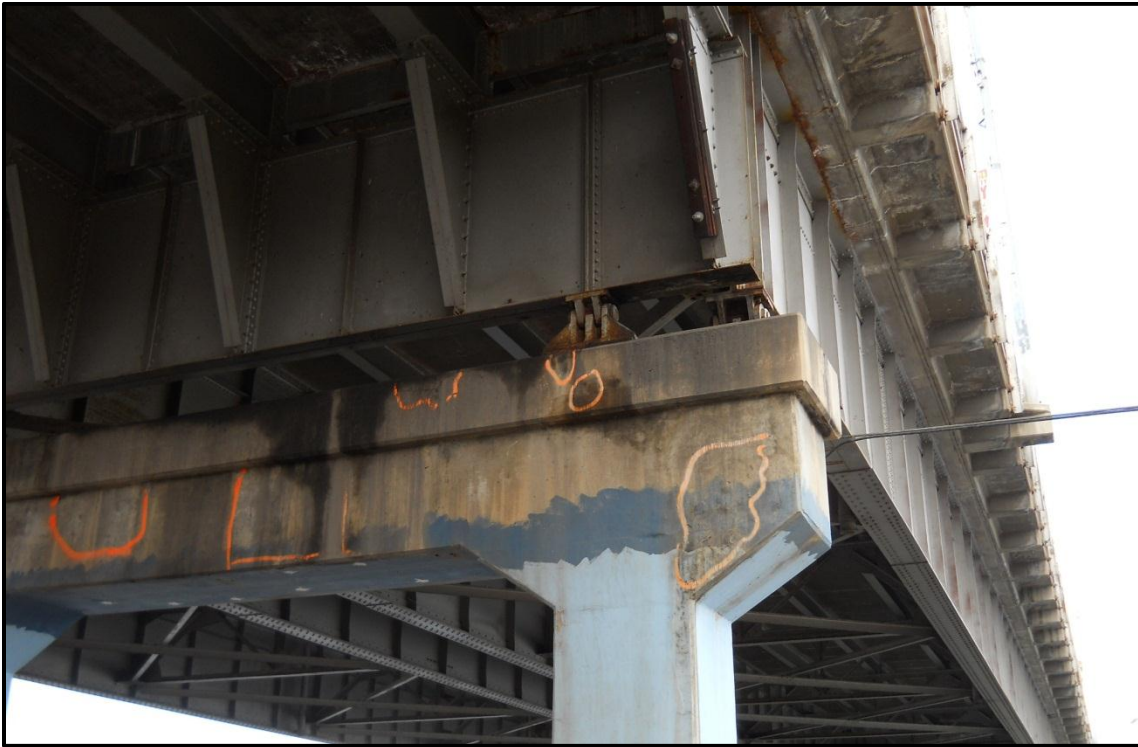
Photo 7. Concrete bent delamination delineated by orange paint and moderately corroded structural steel on the Higgins Avenue Bridge.
