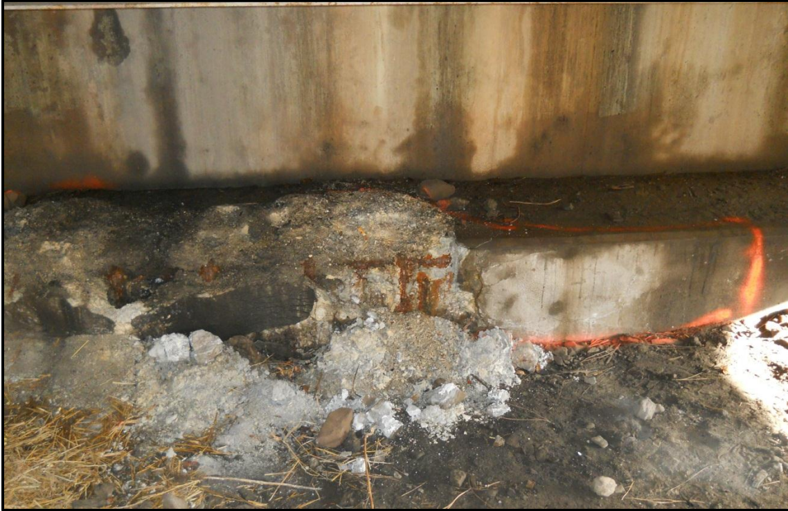
Photo 20. Spalled concrete beam at the north abutment of the Madison Street Bridge
