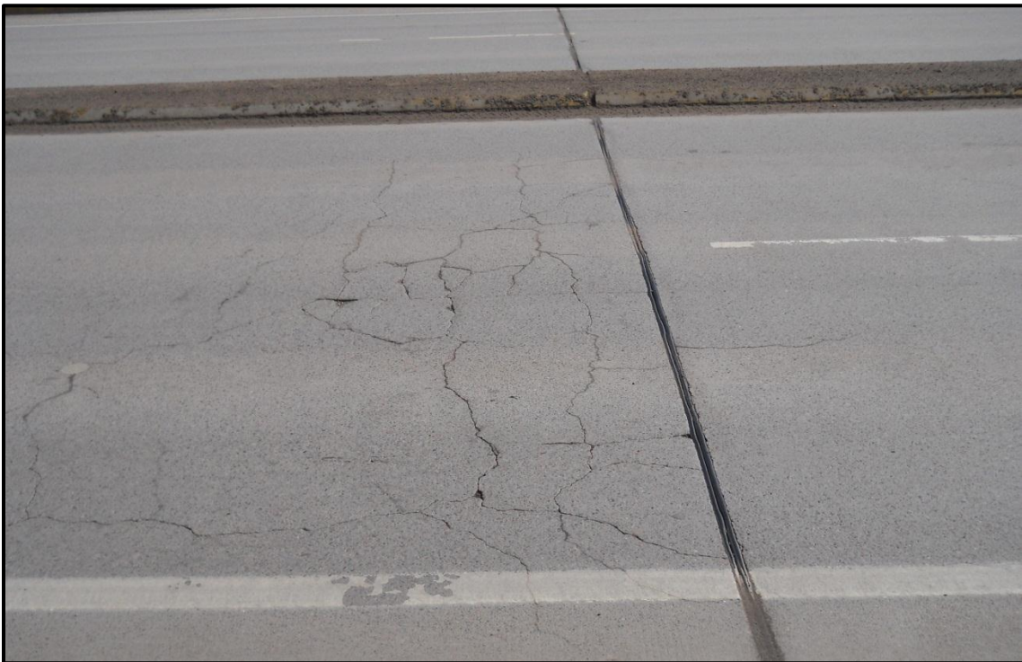
Photo 6. Cracking concrete on the Higgins Avenue Bridge top decking. Photo 5 shows this area from underneath the bridge.
