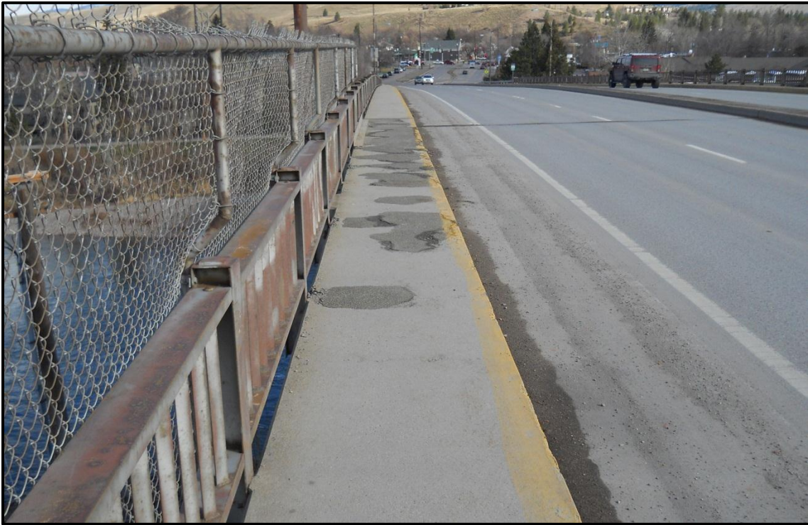
Photo 26. Delaminated and patched sidewalk on the Madison Street Bridge.
