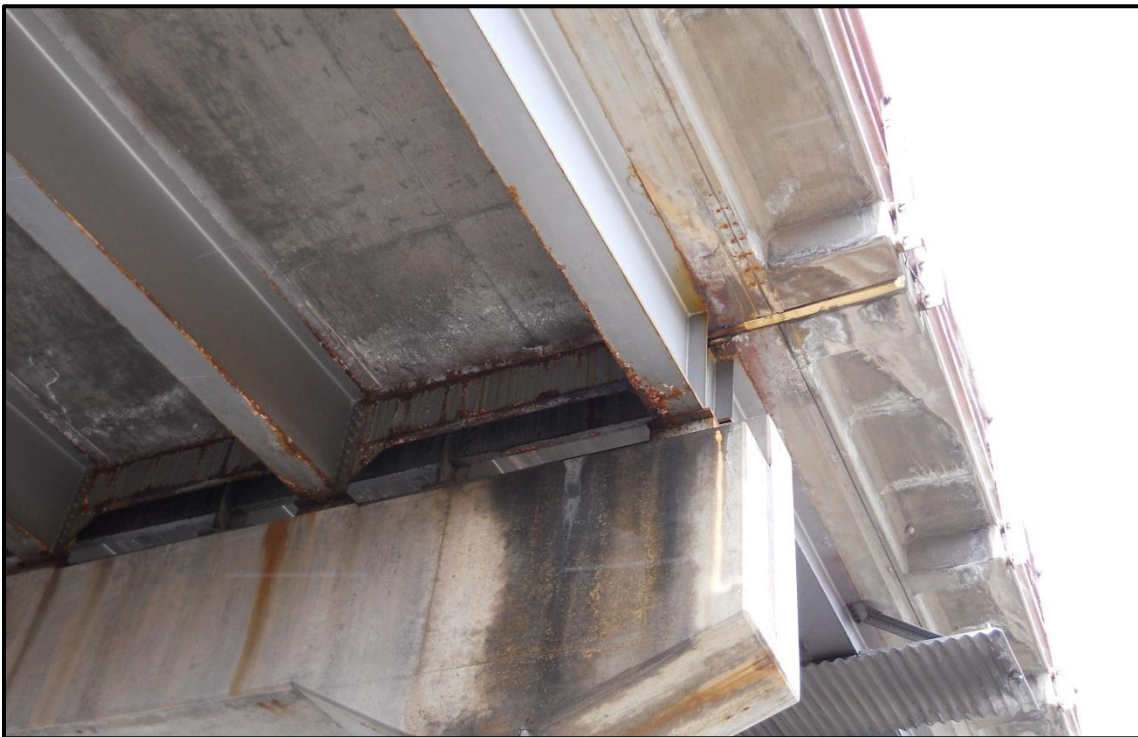
Photo 8. Corroded steel and dark staining of concrete on the Higgins Avenue Bridge.
