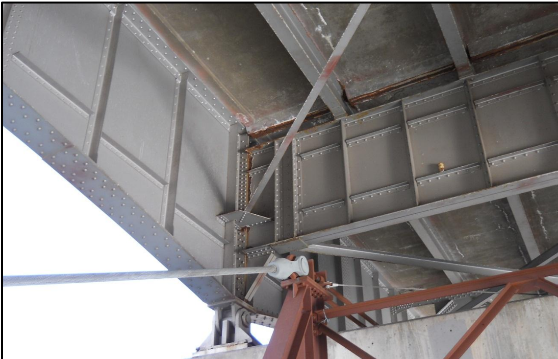
Photo 19. Corroded steel on the Madison Street Bridge.
