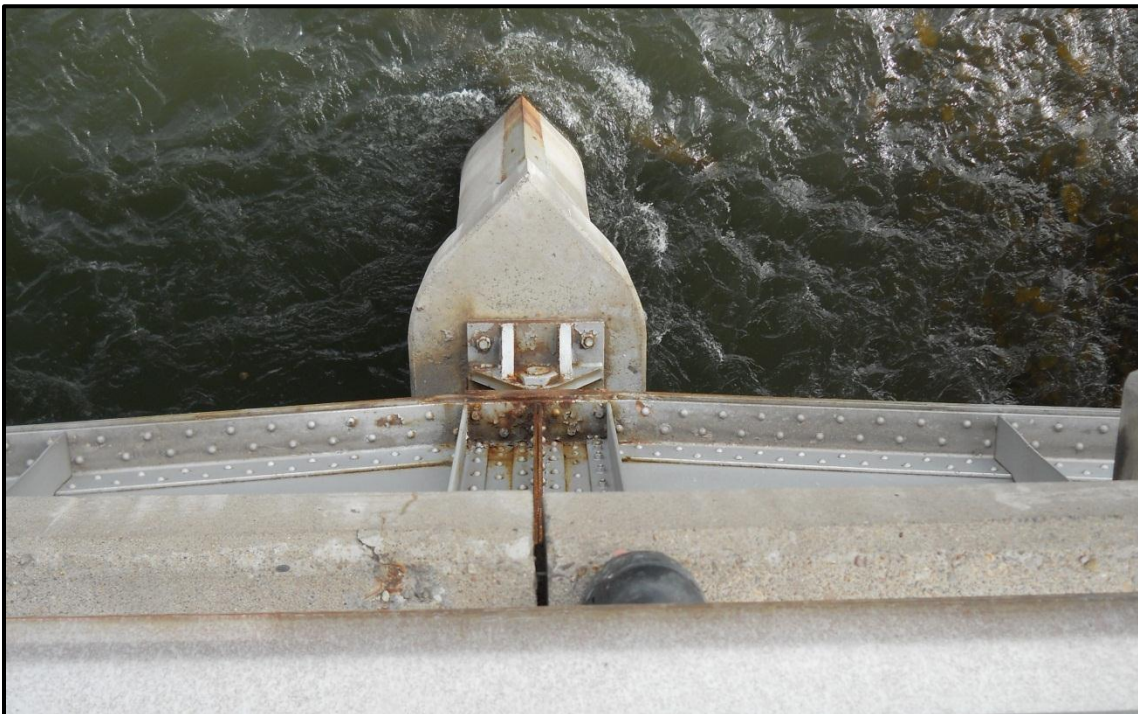
Photo 13. Steel corrosion at a Higgins Avenue Bridge pier and bridge bearing connection.
