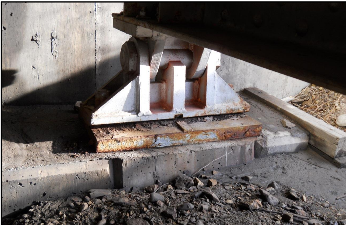
Photo 15. View of girder bearing at the north abutment exhibiting debris/pack rust between the built-up rocker assembly and bearing plate, which may limit the movement of this joint on the Madison Street Bridge.
