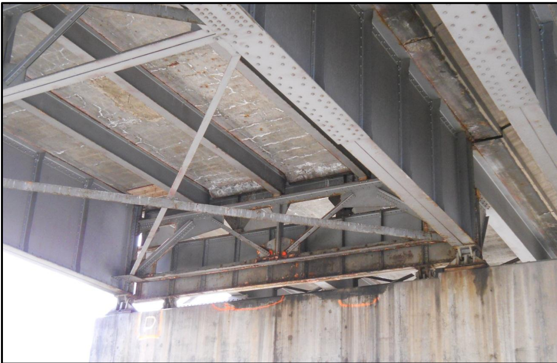
Photo 23. Deterioration of the Madison Street Bridge bent, including corroded steel, cracking concrete with efflorescence, and stains from corroded rebar.
