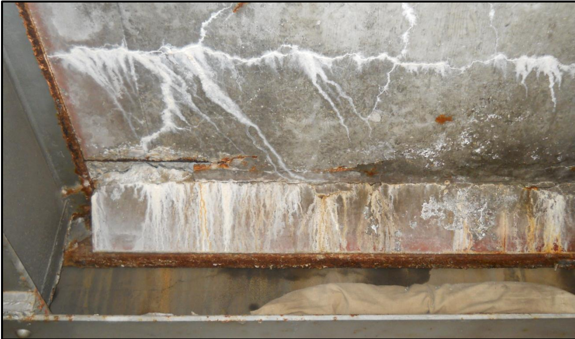
Photo 14. Degradation on the north Madison Street Bridge abutment, including corroded steel, cracking concrete with efflorescence, and concrete staining indicating rebar corrosion.
