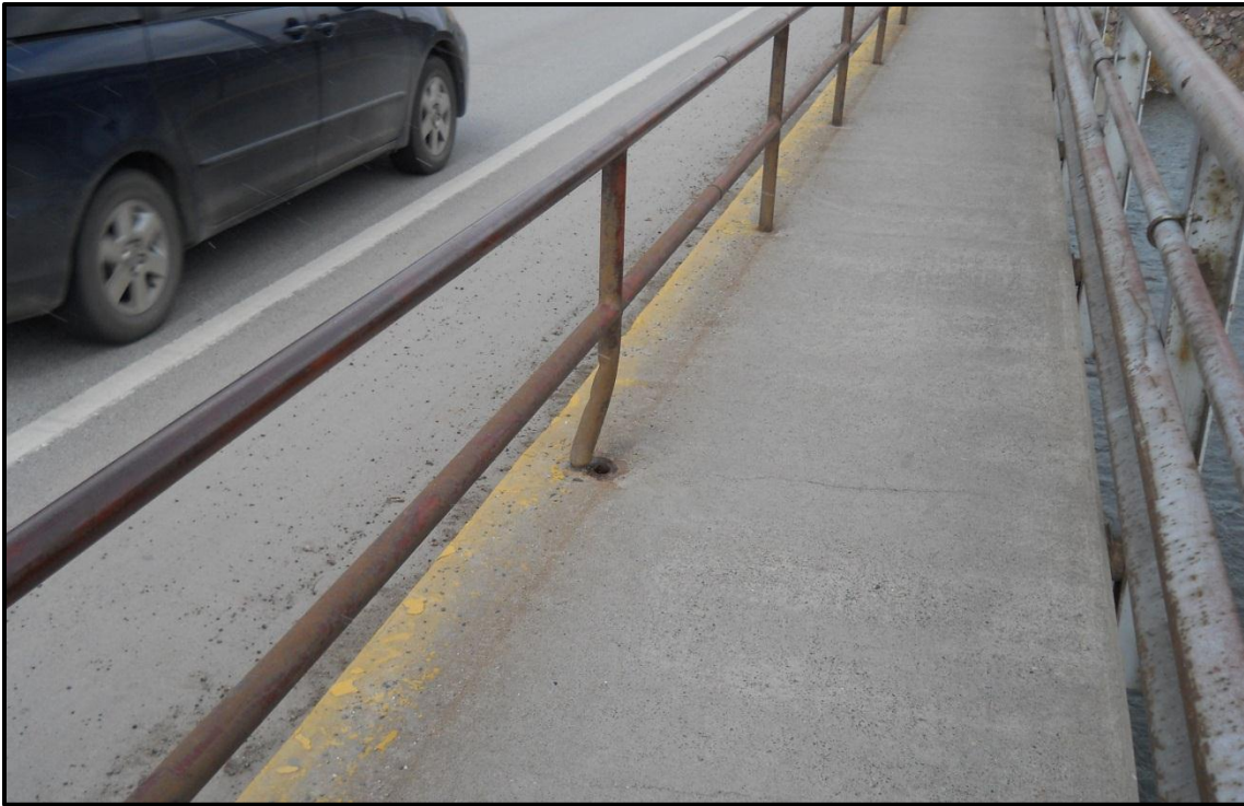
Photo 12. Cracking concrete along the Higgins Avenue Bridge sidewalk and collision damage to the bridge sidewalk railing.
