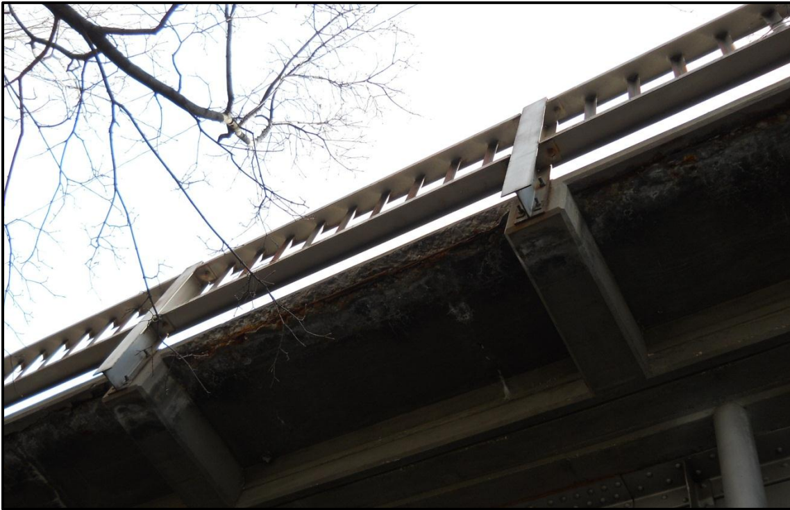
Photo 16. Concrete spalling and corroded rebar at the edge of the Madison Street Bridge. This condition was observed extending over the length of both sides of the bridge.
