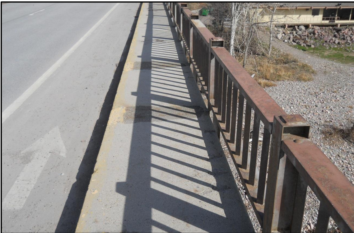
Photo 27. Delaminated and patched sidewalk on the Madison Street Bridge. The railing measures 32 inches in height, which does not meet current standards.
