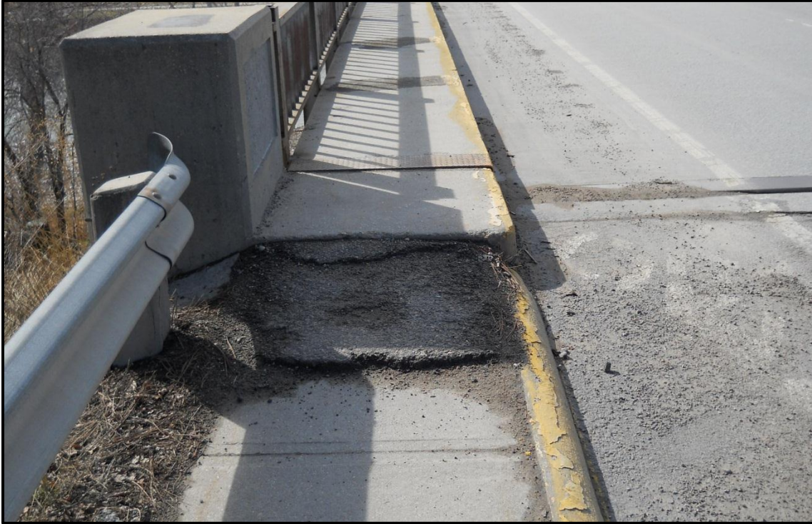
Photo 28. A modified ramp transition area from the roadway sidewalk to the Madison Street Bridge sidewalk. This ramping would not be considered ADA compliant.
