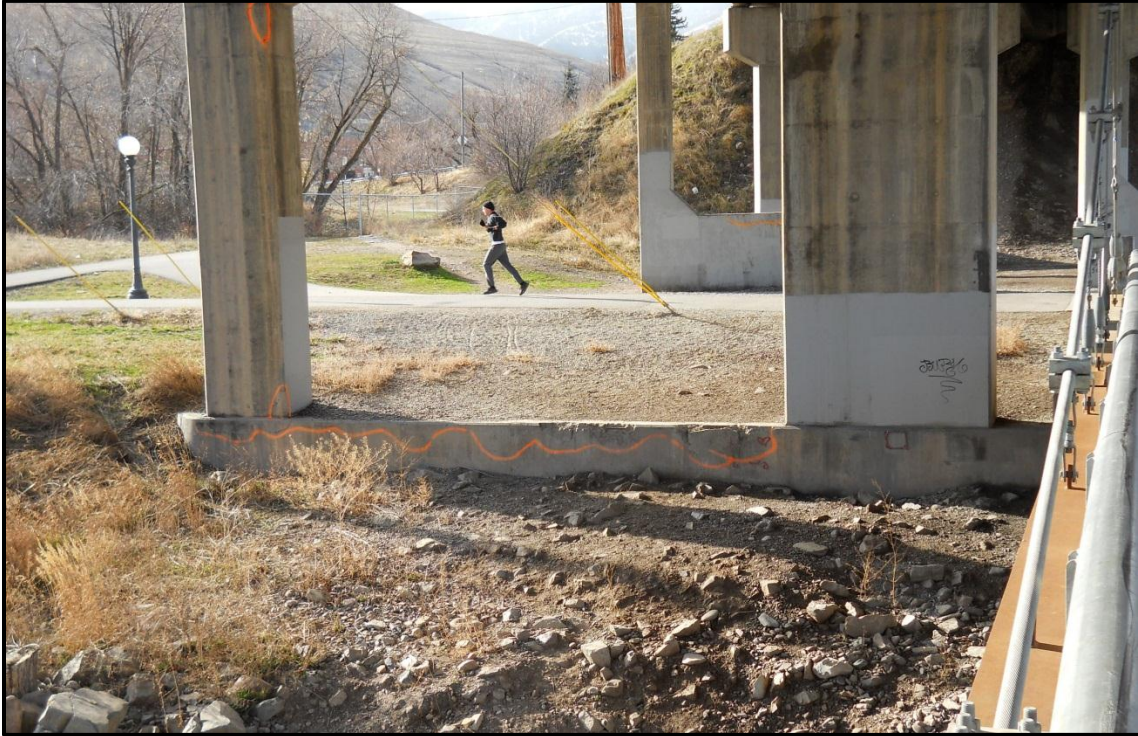
Photo 22. Deterioration of the Madison Street Bridge bent near the ground, including concrete delamination and spalling.
