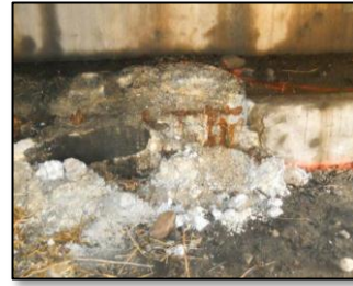
Concrete spalling is a form of surface failure resulting in splintered concrete chips and fragments.
