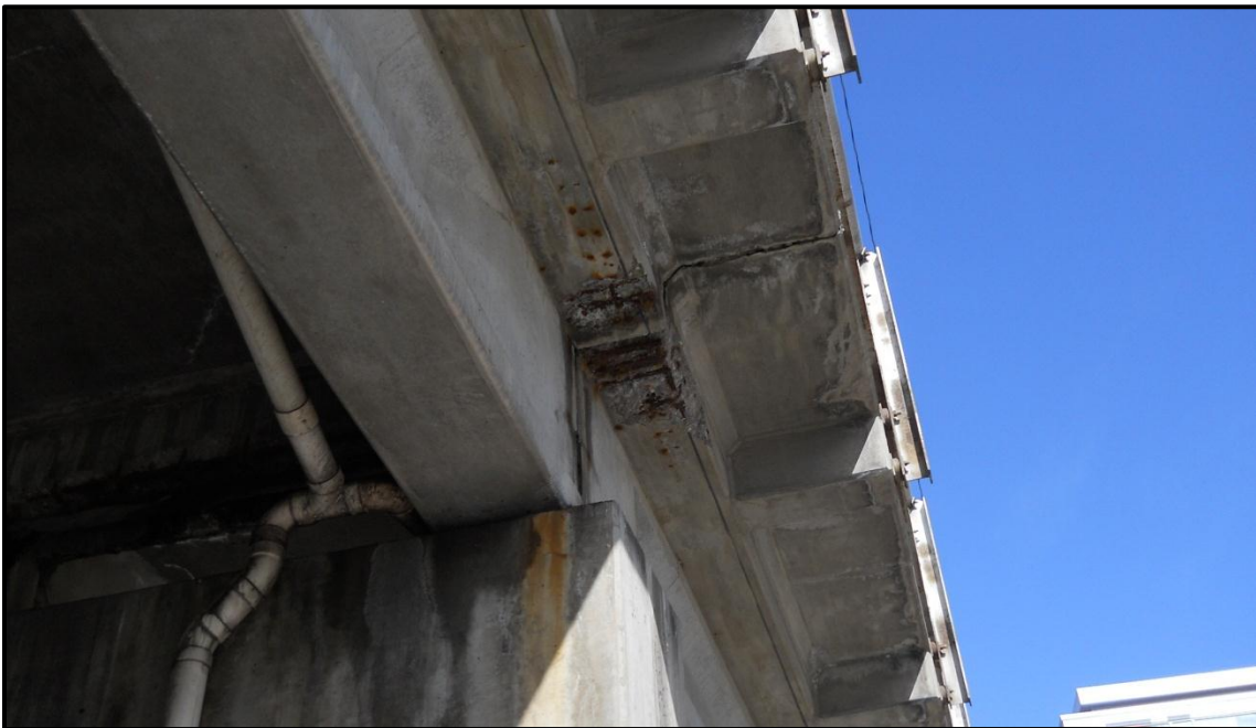
Photo 4. Cracking concrete with efflorescence and steel corrosion on the Higgins Avenue Bridge.
