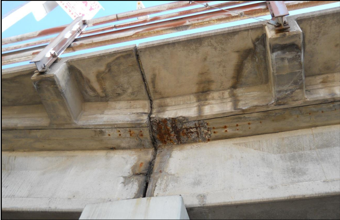
Photo 3. Spalled concrete and corroded rebar in the soffit under the Higgins Avenue Bridge pedestrian sidewalk.
