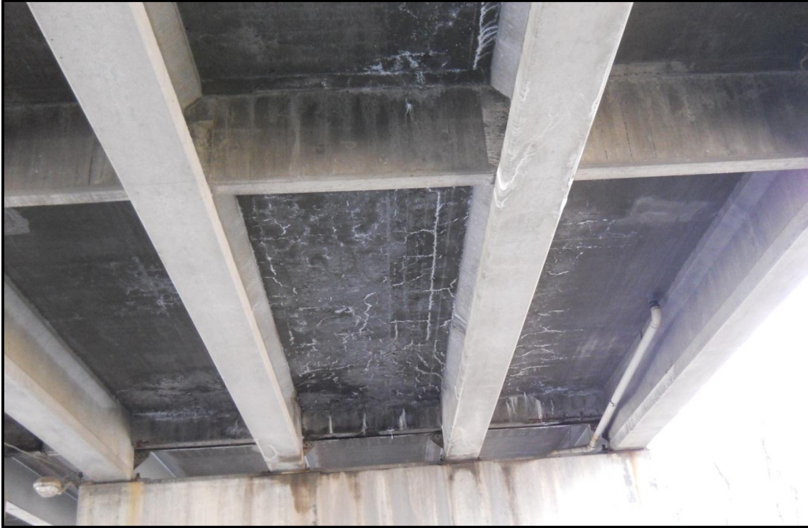
Photo 5. Cracking concrete with efflorescence on the Higgins Avenue Bridge. Photo 6 shows this area from the top side of the bridge.
