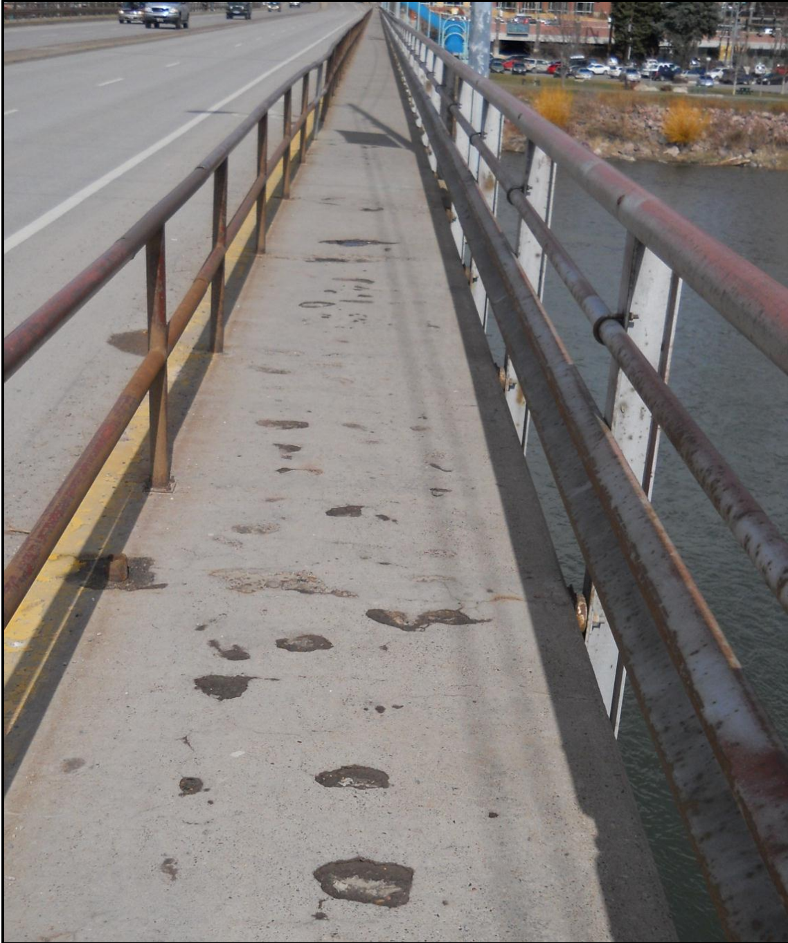
Photo 11. Delamination and spalling concrete along the Higgins Avenue Bridge sidewalk.
