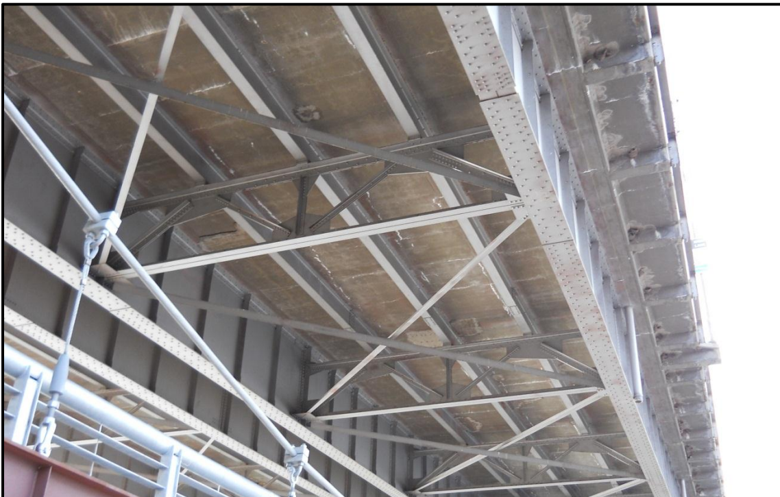
Photo 17. Cracking concrete with efflorescence and patches to concrete sections on the Madison Street Bridge.
