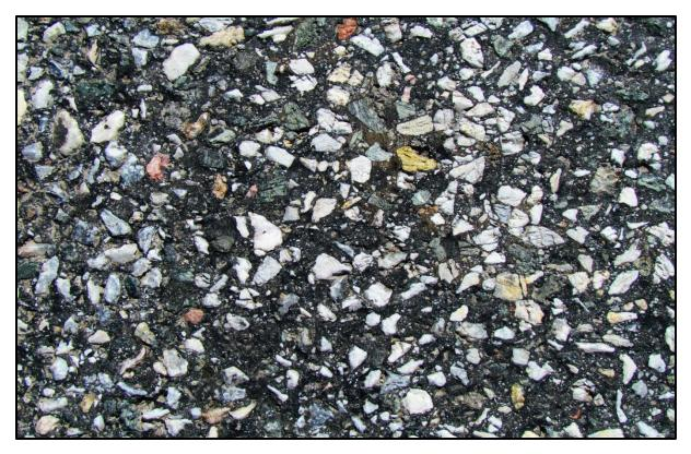
↑ Close-up of typical fog seal over chip seal texture seen in the WB lane.
