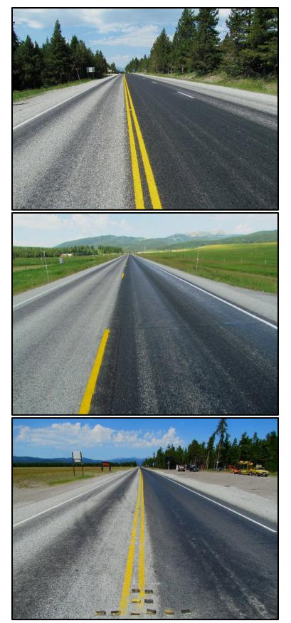
← The following photos were taken several days after fog seal application. CSS-1h emulsion that was factory diluted at a ratio of 50/50 emulsion and water. View west near the Montana/Idaho border.
