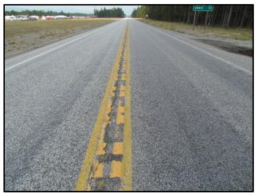
← RP 9.0, view west. The left lane is the chip seal only eastbound lane with the right lane being the fog seal over chip seal westbound lane.
