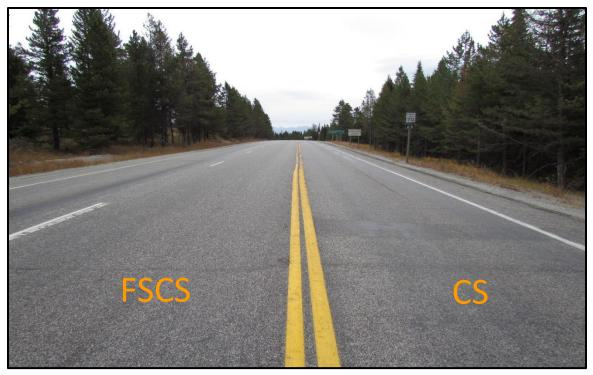
↑ Pavement conditions near RP 0.0 at Montana/Idaho Border, view east. Here the fog seal was not as visible compared to the other end of the project, seen below.
