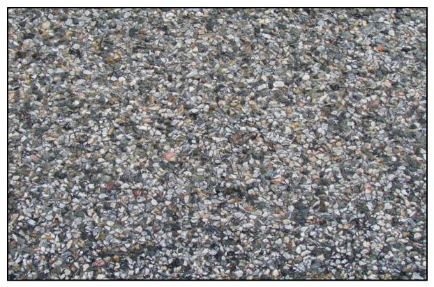
↑ Close-up of the typical chip seal texture seen in the EB lane (control).
