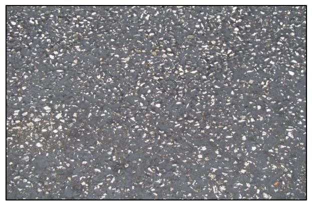
↑ Close-up of the typical fog seal over chip seal texture seen in the WB lane (test).
