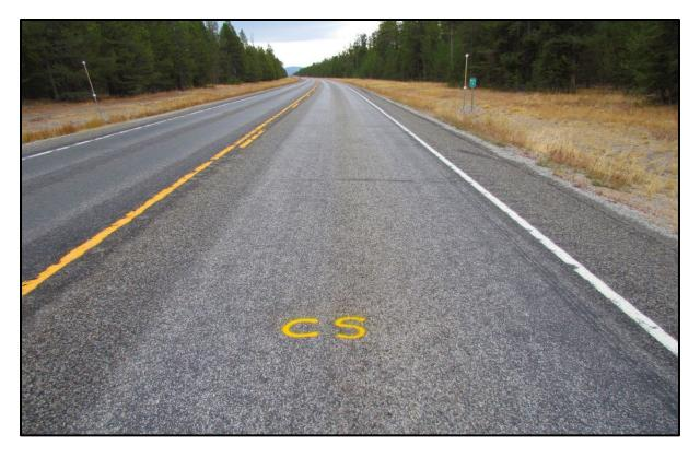
♠♥ Comparison of the EB chip seal (above) and WB fog seal over chip seal (below) near RP 5.0, view east.
