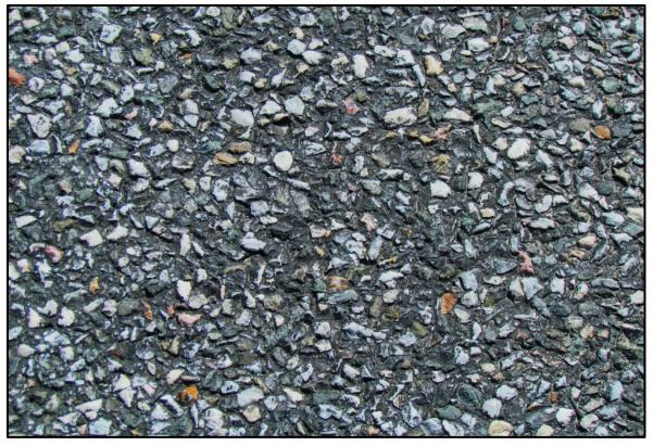
↑ Close-up of texture of fog seal on seal and cover (FSCS).
