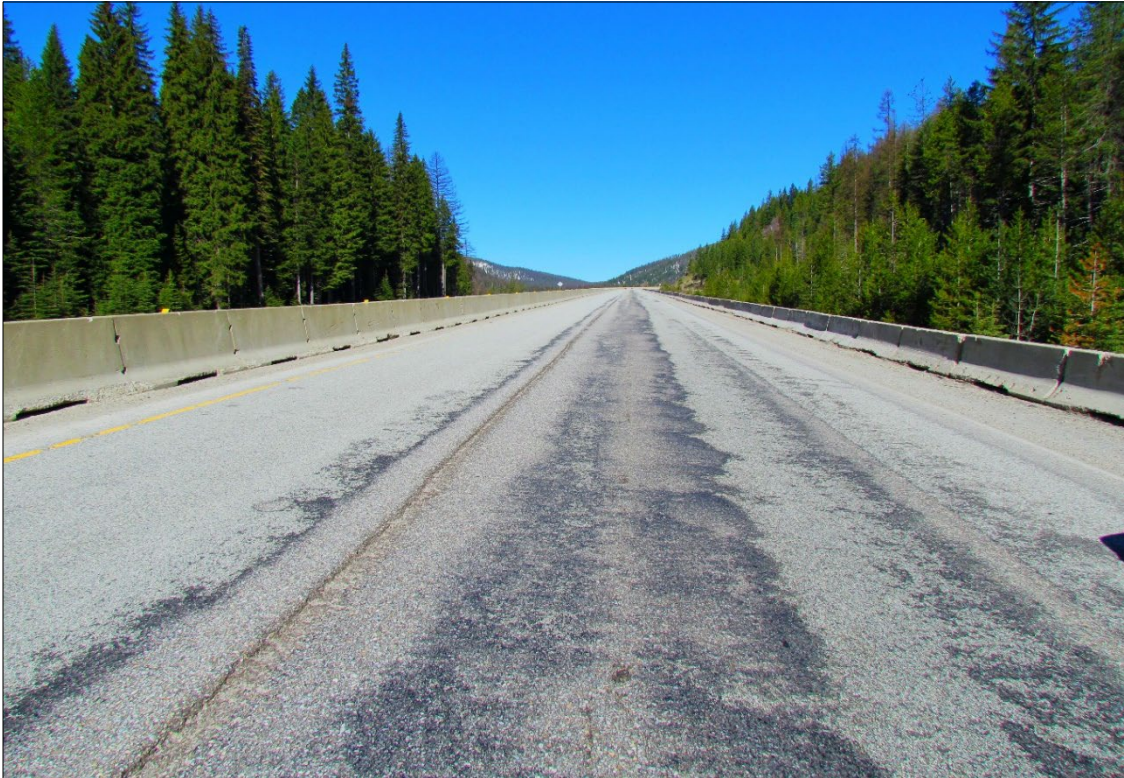
↑ FSCS section; view west.
