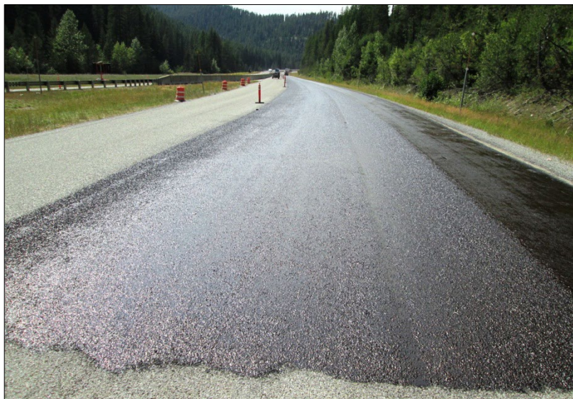
↩️ Completed pass of FSCS emulsion.
