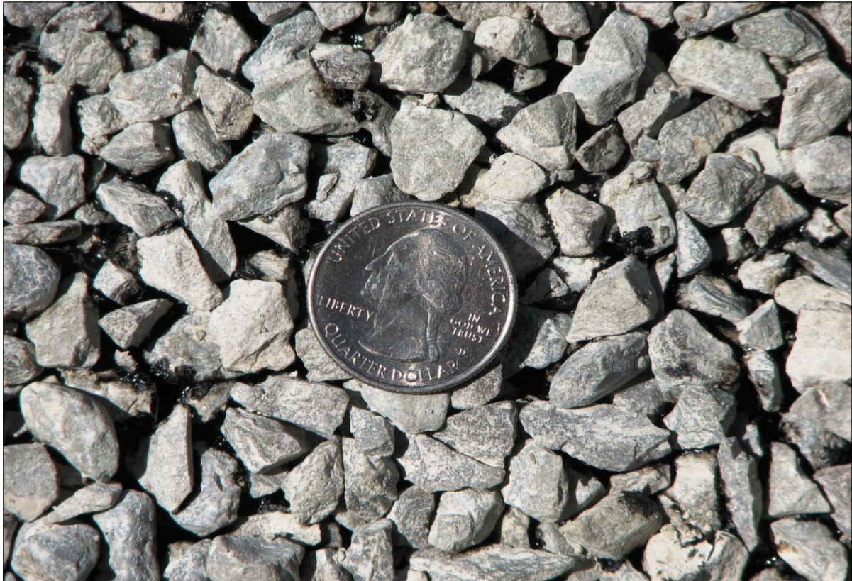
↑↓ Average visual appearance of chip seal embedment on project after cure and sweeping phase completed.
