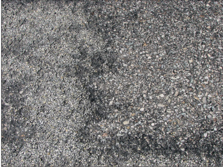
← Example section of FSCS removed to asphalt surfacing.
