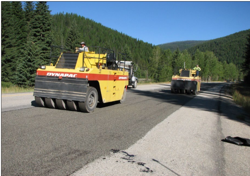
← Several nine-tire pneumatic rollers are used in the compaction phase.
