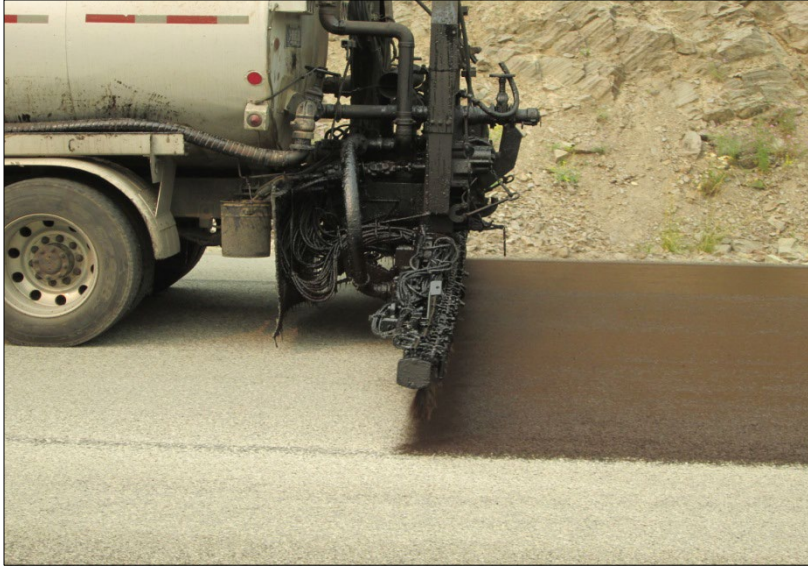
↩️ The CSS-1 Emulsion was applied at a diluted rate of 50/50 in one pass.
