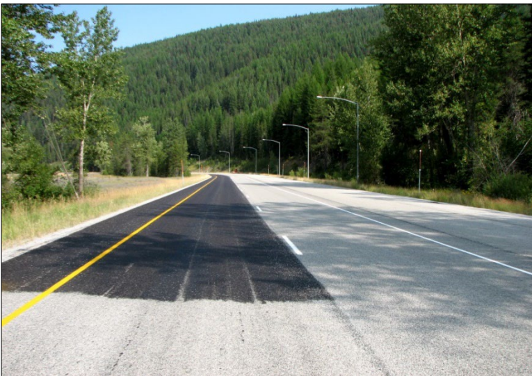
← Extended Section of FSCS at approximate reference point 3.5; westbound passing lane.
