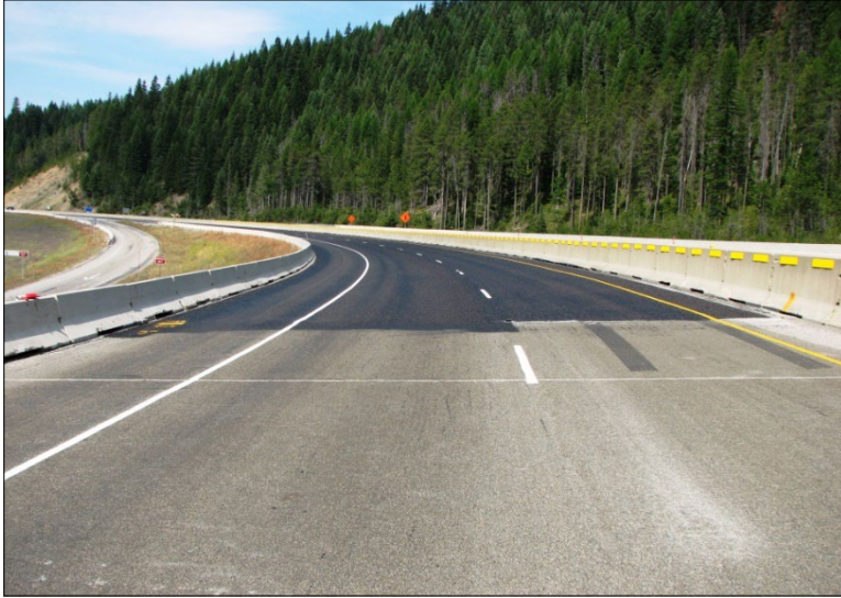
← Section of eastbound FSCS at approximate reference point 5.7/Taft Area Interchange: View west.
