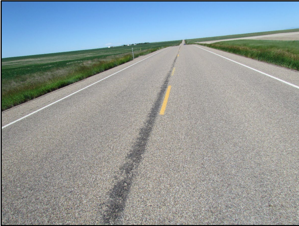
↑ View of centerline chip loss near RP 361.
