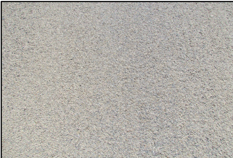
←↓ Several images of embedded chip texture.
