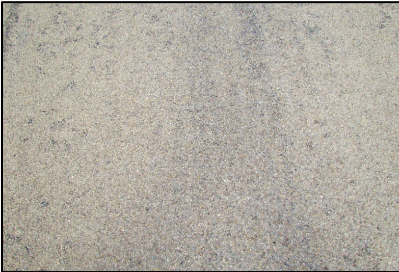
←↓ Several images of embedded chip texture.
