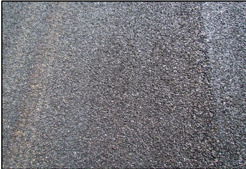
←↓ Several images of fog seal and chip texture.
