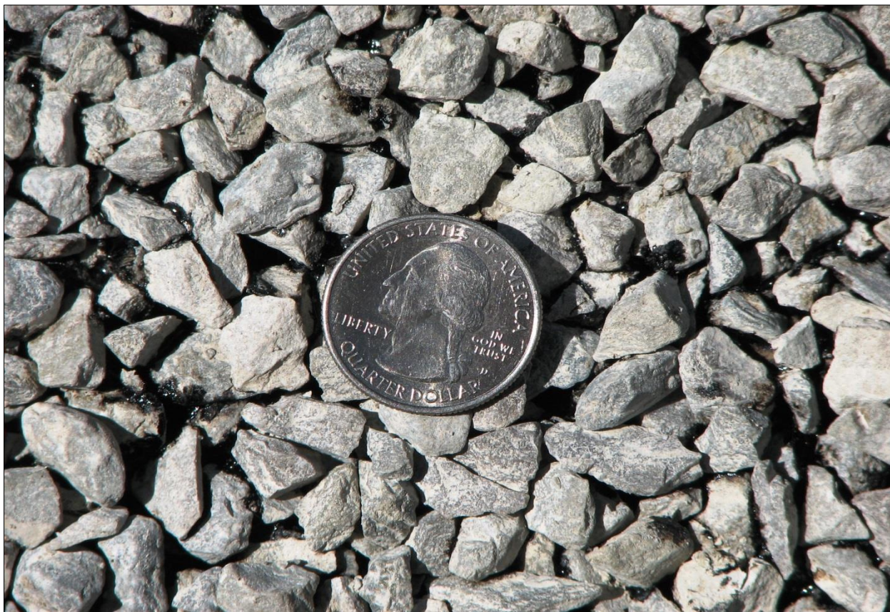
↕ Average visual appearance of chip seal embedment on project after cure and sweeping phase completed.
