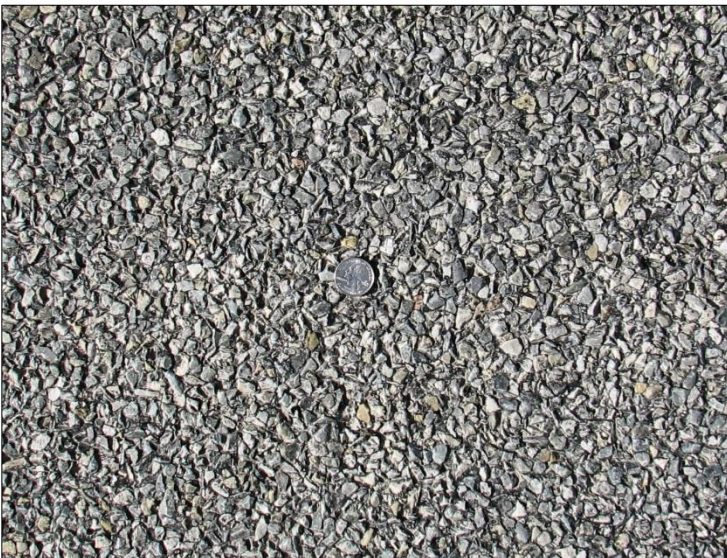
← Close-up of intact FSCS surface texture.
