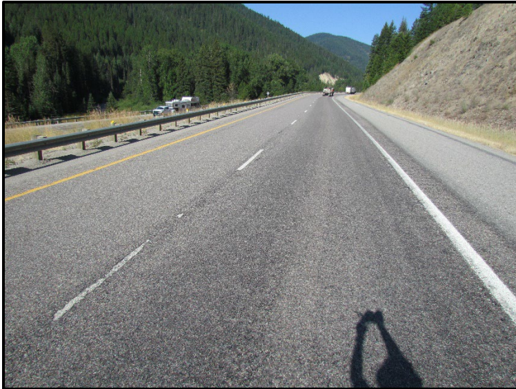
← RP 12, westbound, view west.
