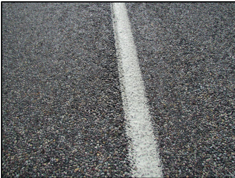
← RP 12, close-up view of the chip seal condition at the fog line.
