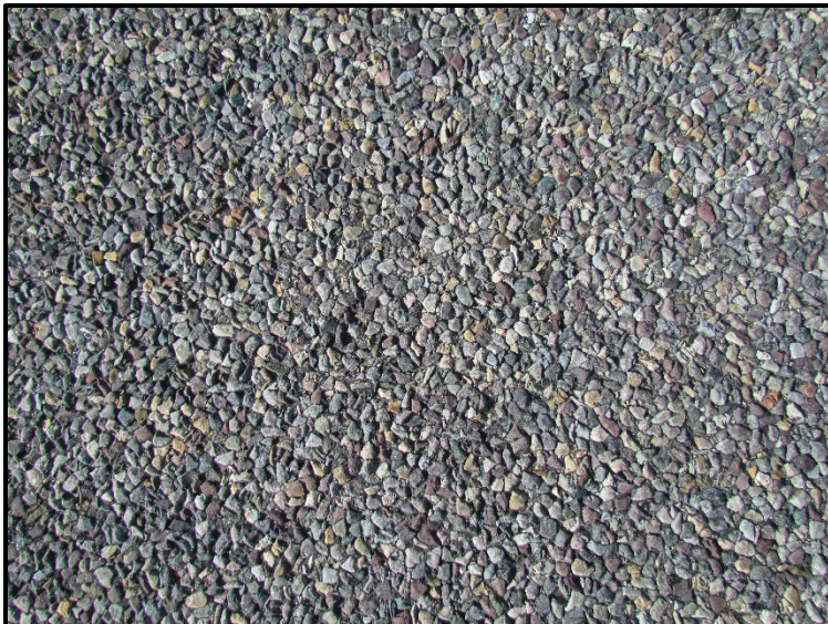
← RP 12, close-up of the chip seal surface.
