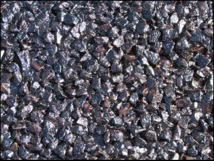
← Close-up of completed FSCS application with CSS-1h emulsion.
