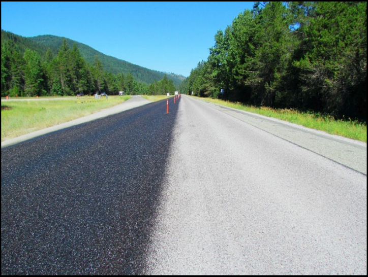
← Representative image of FSCS application in progress.
