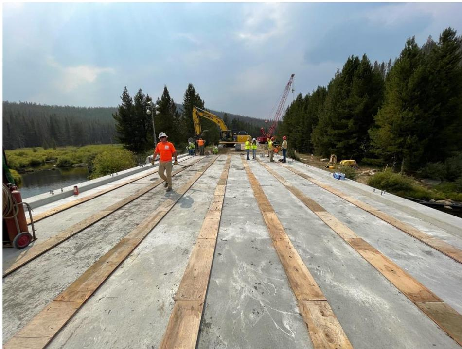
Figure 5: Keyways with top forming
