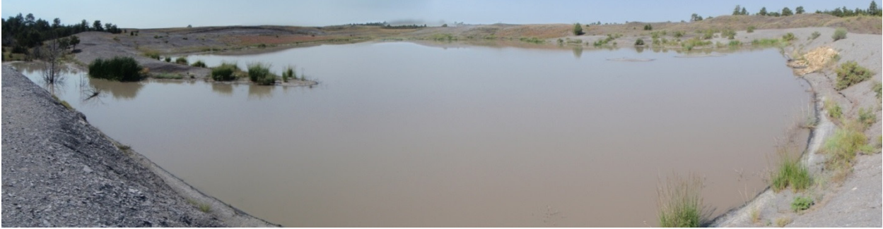
Photo Point 2; Location: NE edge of wetland cell; Bearing 230 degrees; Year 2013
