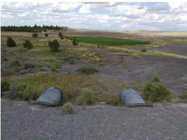
Photo Point 5 Location: Outside North Border Bearing: 10 degrees Year 2016
