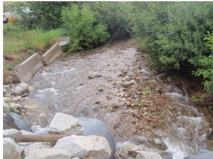
Photo Point 12 – Photo 1 Location: Upstream of culvert Bearing: South Taken in 2012
