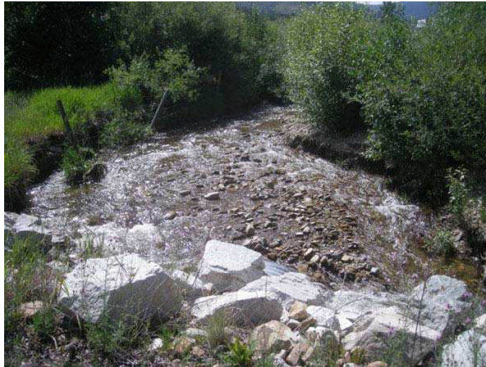
Photo Point 12 – Photo 1 Location: Upstream of culvert Bearing: South Taken in 2009
