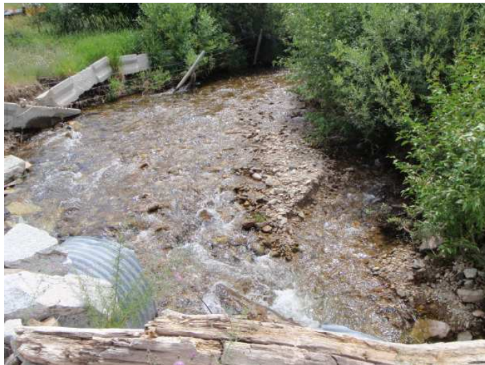
Photo Point 12 – Photo 1 Location: Upstream of culvert Bearing: South Taken in 2011
