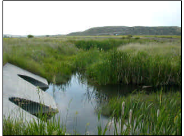
Location: K Description: Outlet of #1 Compass Reading: SE
