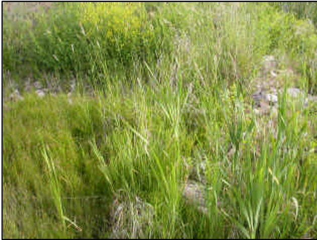
Location: J Description: Rip rap to #2 Compass Reading: N
