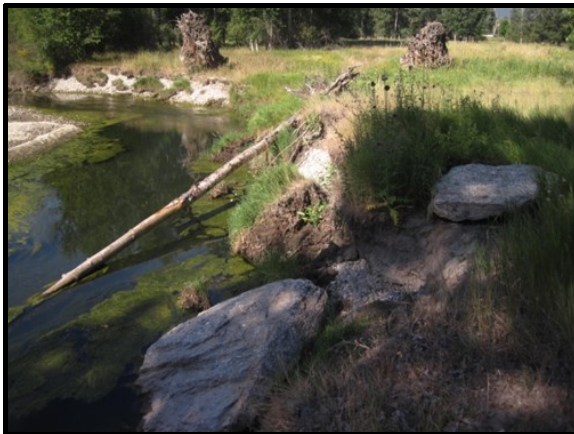
Photo Point 4.4: View of boulders, logs, and root wads placed on bank. Compass: 248 (West-Southwest)
