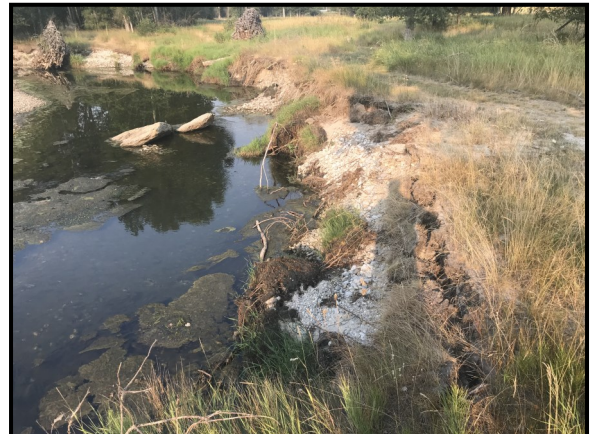
Photo Point 4.4: View of boulders, logs, and root wads placed on bank. Compass: 248 (West-Southwest)
