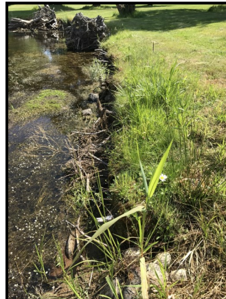
2013 Photo Point 2: View of un-keyed coir log on south bank. Compass: 90 (East)
