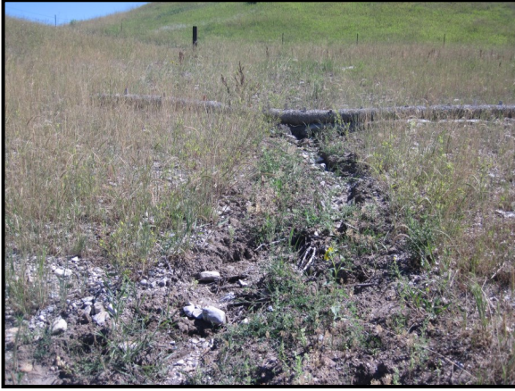
Additional Photo 5: Gully identified along east site of reconstructed channel
