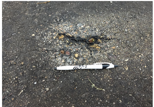
T-3, Swell and Mechanical Raveling
