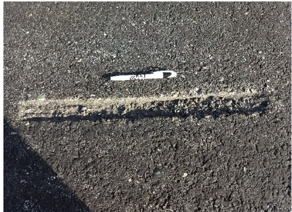
R-2, Routed Crack with Sealant
