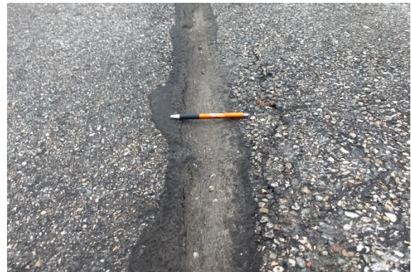
A-11, Crack Sealed
