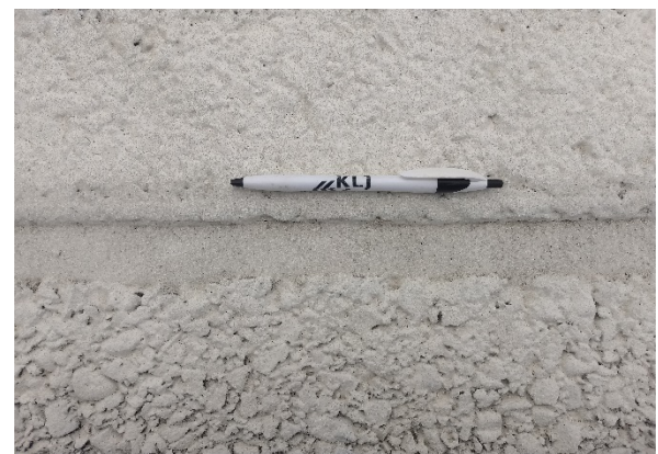
R-11, Sealed Crack
