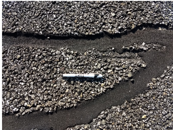
R-2, Cracks
