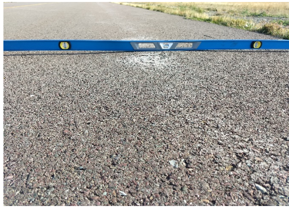
T-2, Swell and Mechanical Raveling
