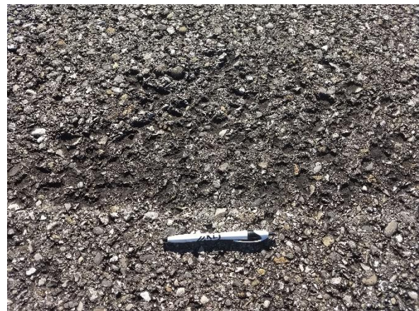
T-2, Mechanical Raveling
