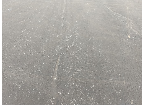
A-2A, Cracks
