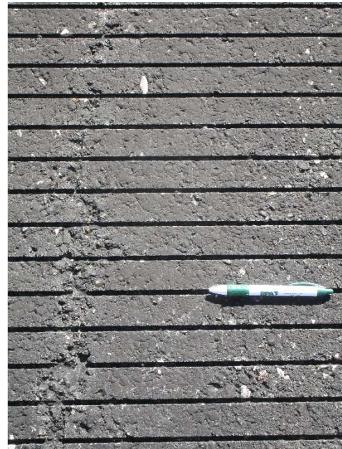
R-2, Surface detail with raveling
