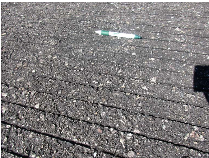
R-1, Surface detail with weathering & raveling
