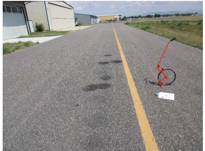
T-4, Overview with oil spills
