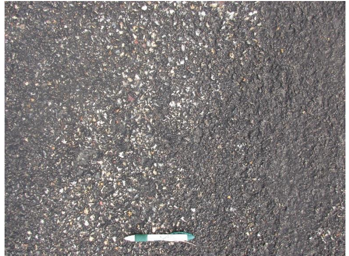
T-11, Surface detail with scraping
