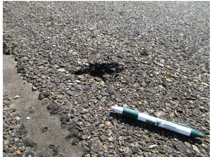
A-3A, Surface detail with raveling
