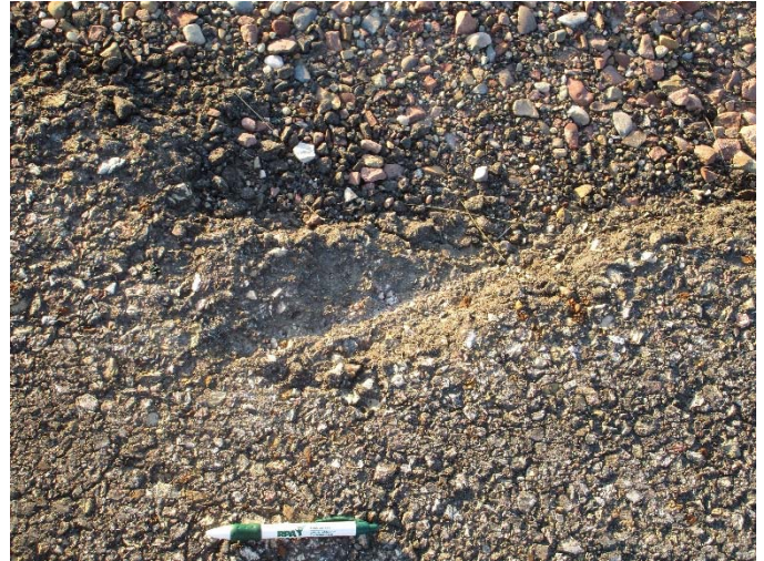
T-17, Surface detail with gouging
