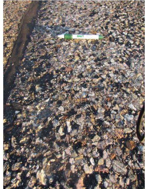
T-22, Surface detail of gouge / ravel
