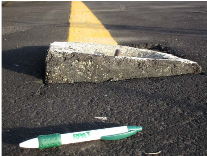
A-11 , Surface detail with displaced tie down
