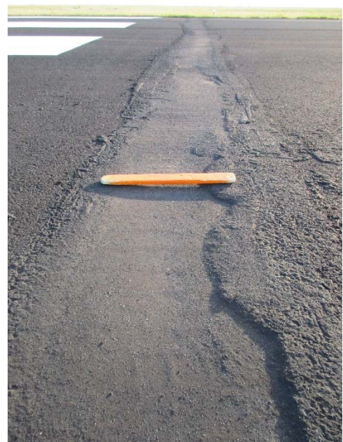
R-11 , Surface detail with patching
