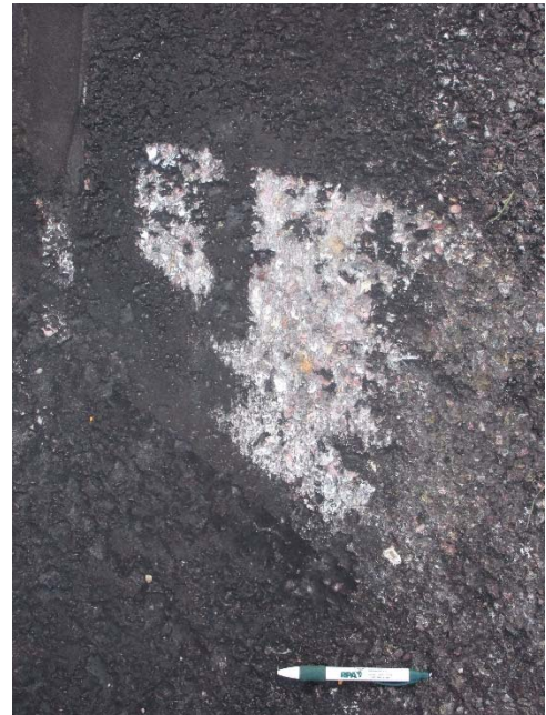
A-11, Surface detail with scrape / raveling
