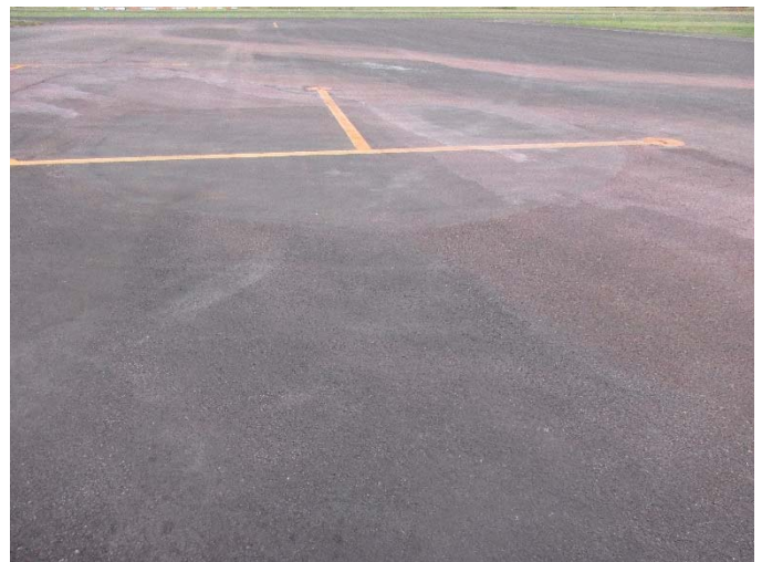
A-12, Overview with fire retardant stains
