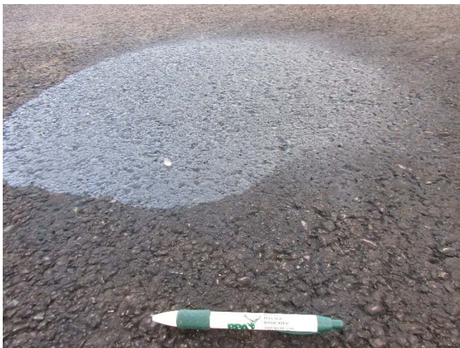
A-12, Surface detail with oil spill
