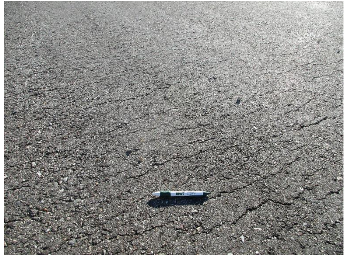
T-5, Surface detail with roller checking
