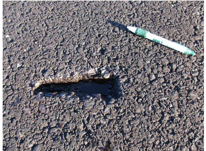
A-11 , Surface detail with gouge
