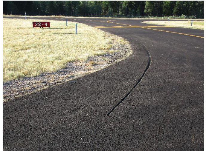
T-11, Surface detail with large gouge
