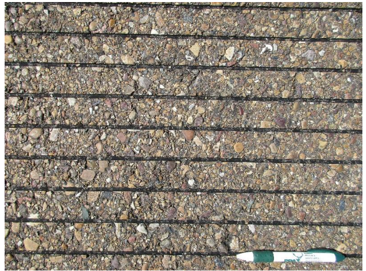
R-13, Surface detail with grooves
