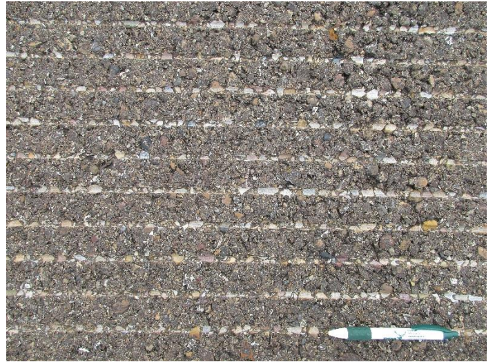
R-15, Surface detail with grooves
