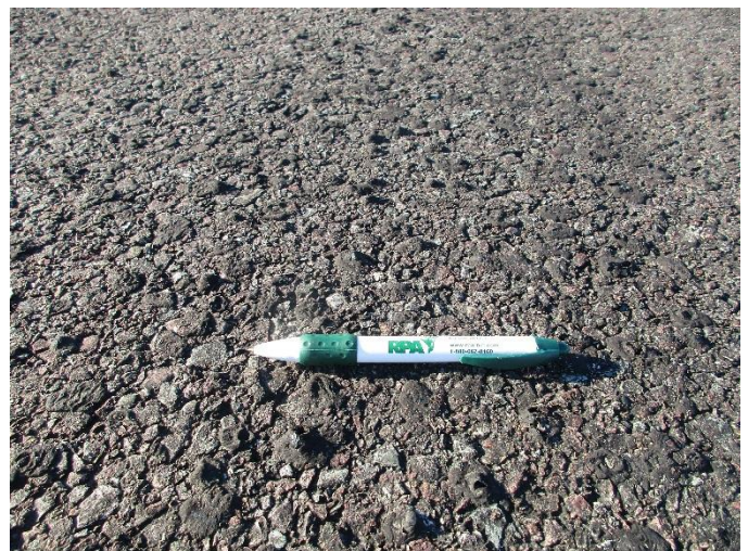
T-3, Surface detail with minor bleeding
