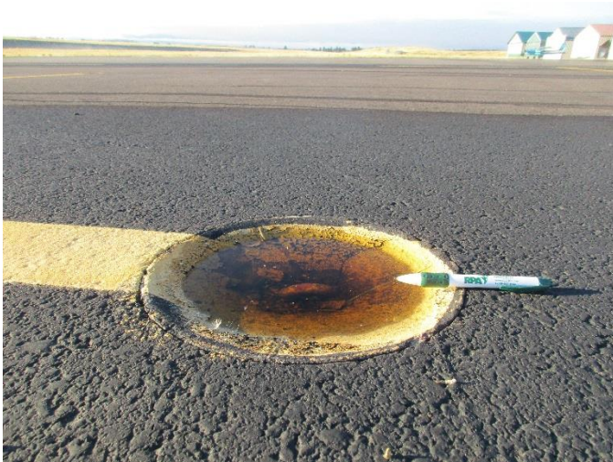
A-1 , Surface detail with tie down
