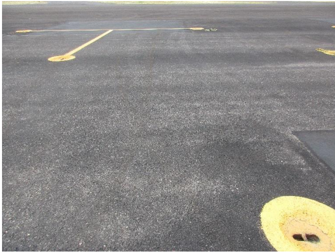
A-3, Overview with tie downs
