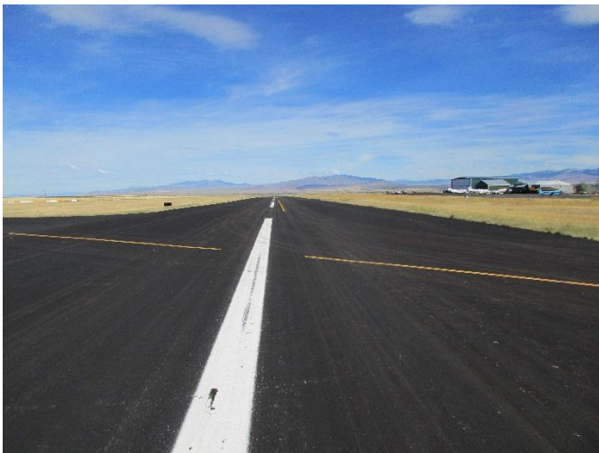
R-3 , Striping overview
