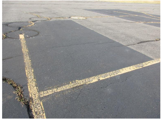
A-1 , Overview with patching
