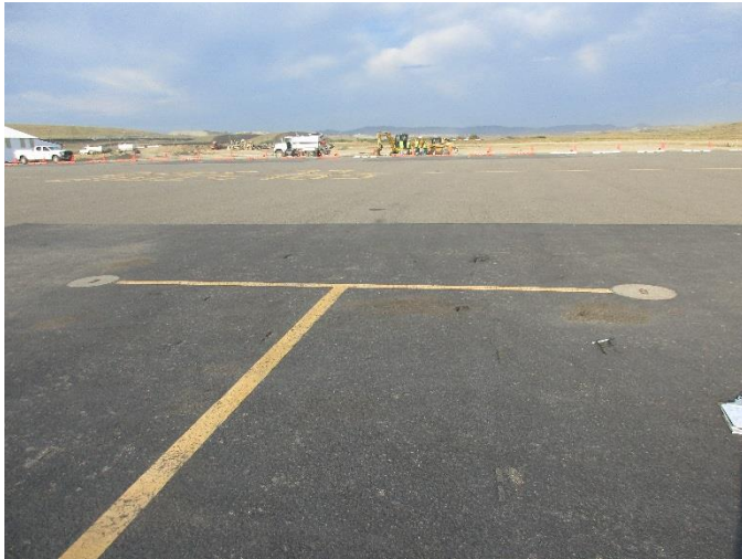
A-1 , Overview with tie downs
