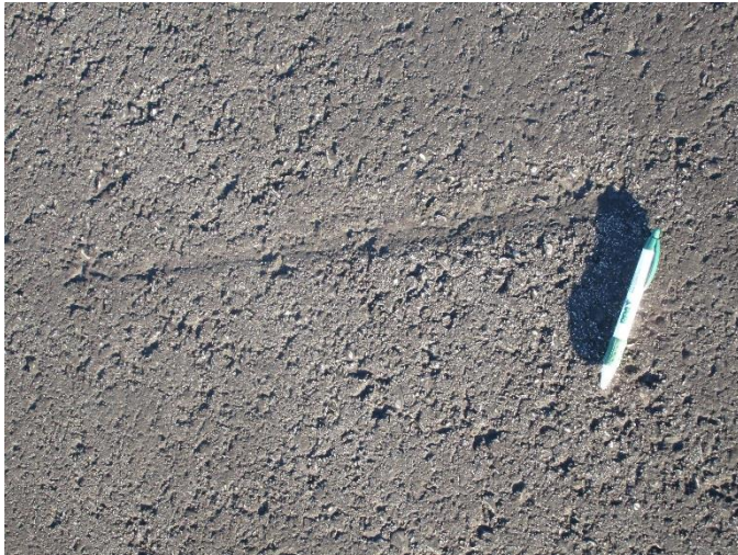
T-2 , Surface detail with gouge
