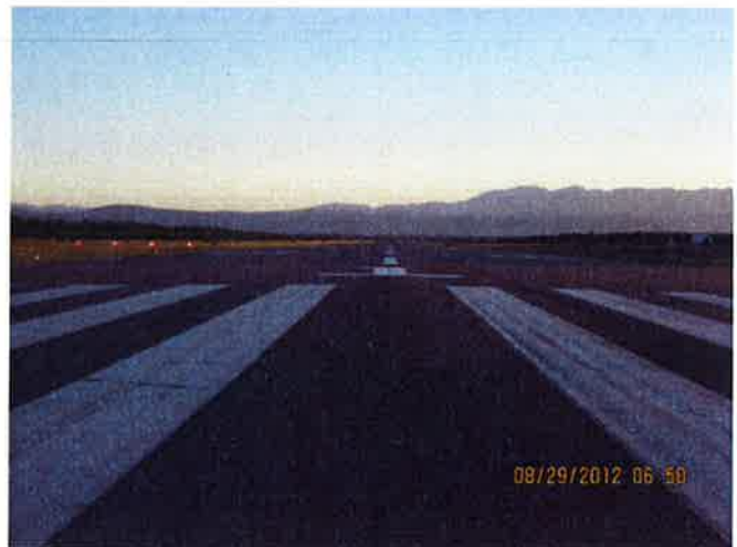
R-2, South overview
