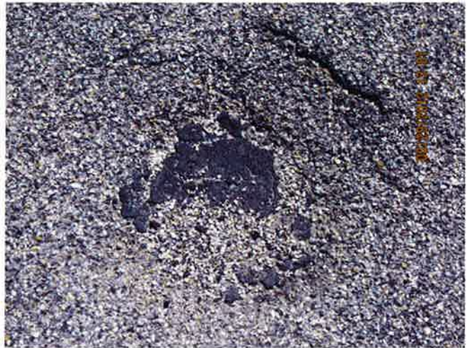
T-1, Surface detail with depression
