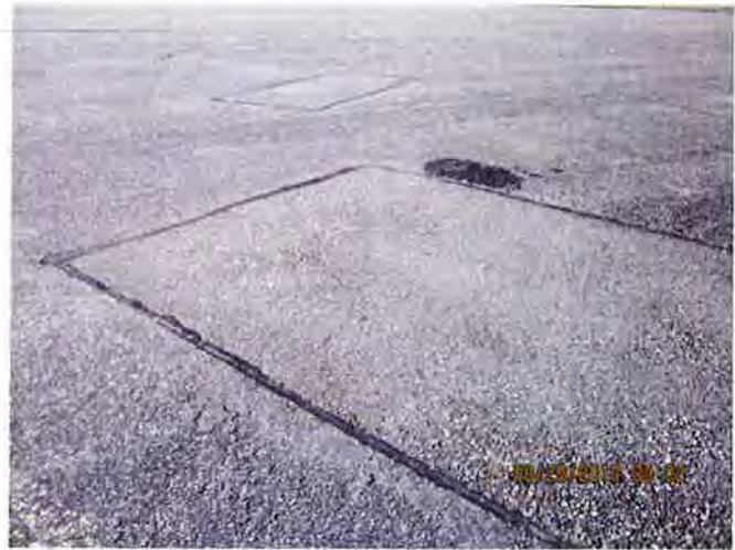
A-3, Surface detail patching
