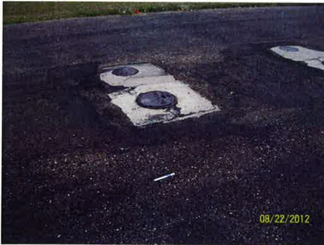
A-11, Overview over underground tanks
