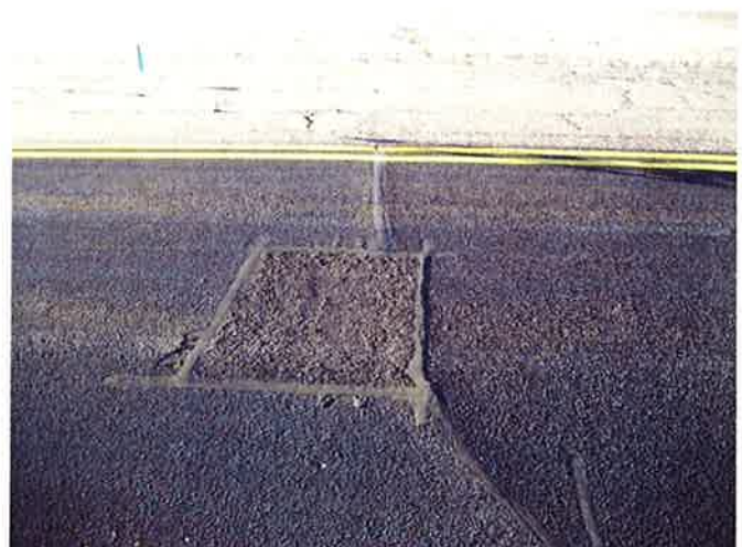
T-4, Surface detail patching
