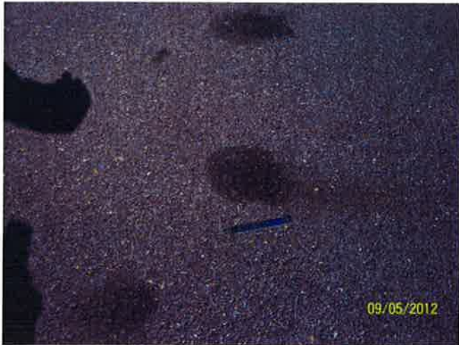
A-1 , Oil spillage
