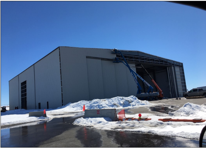
Hangar construction as of March 2019
