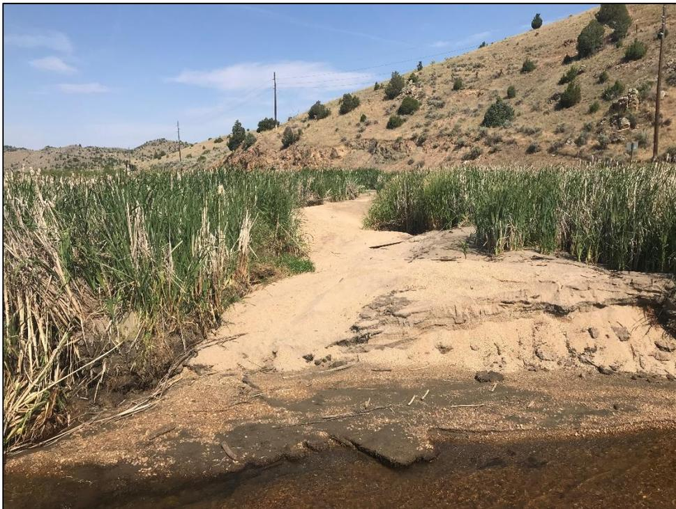
*Photo 4. Sediment deposits adjacent to Granite Creek immediately downstream of Highway 287 Bridge.*
