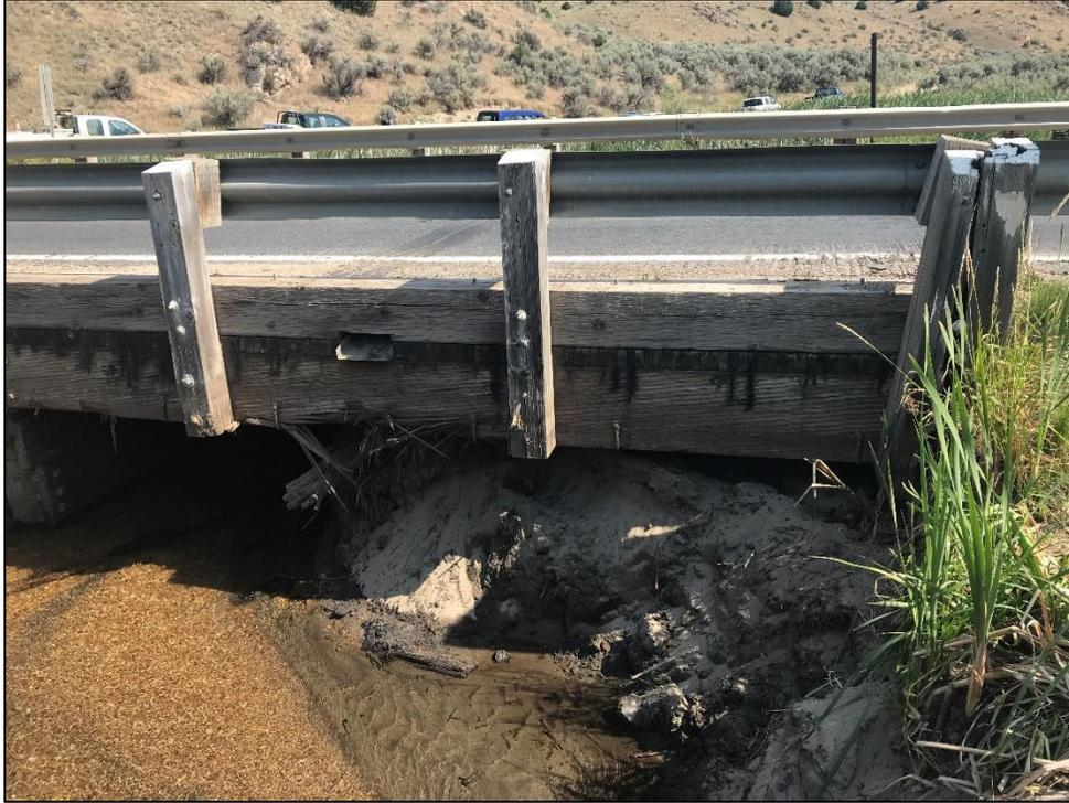
*Photo 3. Fine gravel, sand, and silt deposits beneath Highway 287 Bridge over Granite Creek.*
