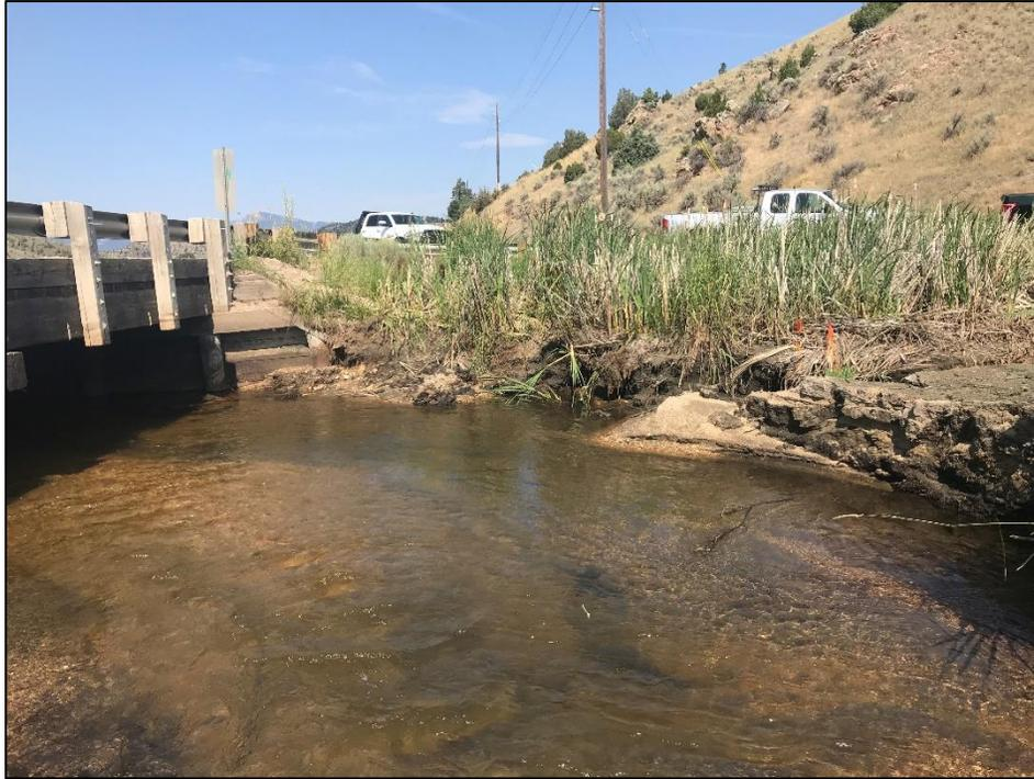
*Photo 1. Sediment deposition observed on upstream side of Highway 287 Bridge over Granite Creek*
